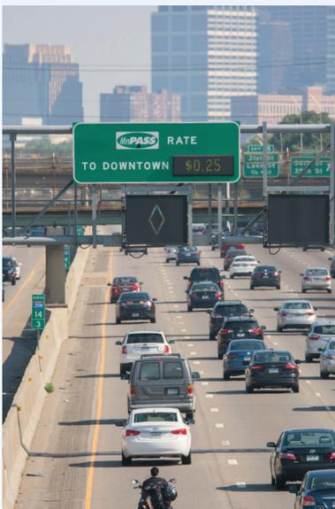
A PDSL automatically changes status based on traffic conditions. The diamond indicates that it is open as a high-occupancy-only lane.
