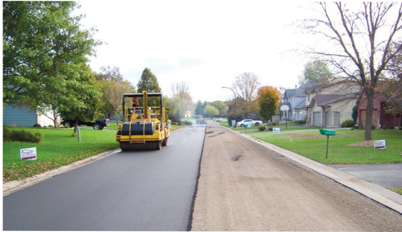
Compacting and smoothing pavement is one of the last steps in FDR of urban and suburban roads. FDR has been shown to be more cost-effective than standard mill-and-overlay approaches.
