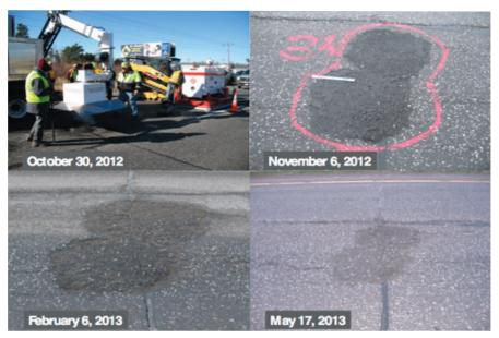
The truck-mounted microwave unit (top left) heated both the pavement and the new patching material made from Minnesota taconite mining byproducts, creating a durable bond between pavement and fill. The repair was then monitored over several months.
