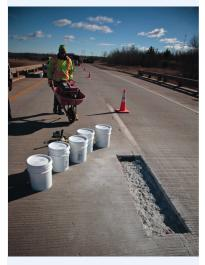
Under the right conditions, taconite-based Rapid Patch can be mixed in and poured from a bucket or a wheelbarrow to repair concrete pavements.
