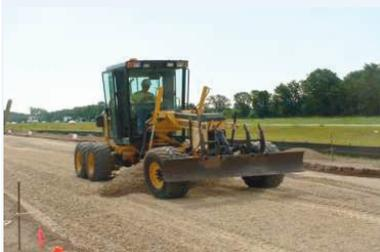
Open graded aggregate bases have improved drainability and similar structural stability to traditional dense graded base layers.
