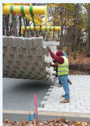
Permeable interlocking concrete pavers like these can be installed fairly quickly.
