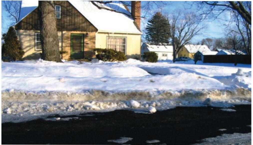
Even with little or no road salt, a permeable pavement like this porous asphalt in Robbinsdale, Minnesota, collects little slush and snow in the winter because it warms well and remains porous enough to infiltrate surface water effectively.
