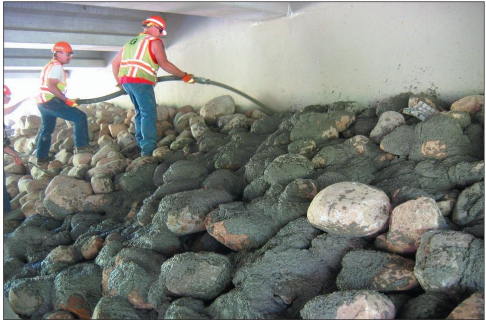
Grout was applied to riprap underneath a bridge in Milaca, Minnesota, creating a stronger scour countermeasure with more rounded rocks than typical riprap.
