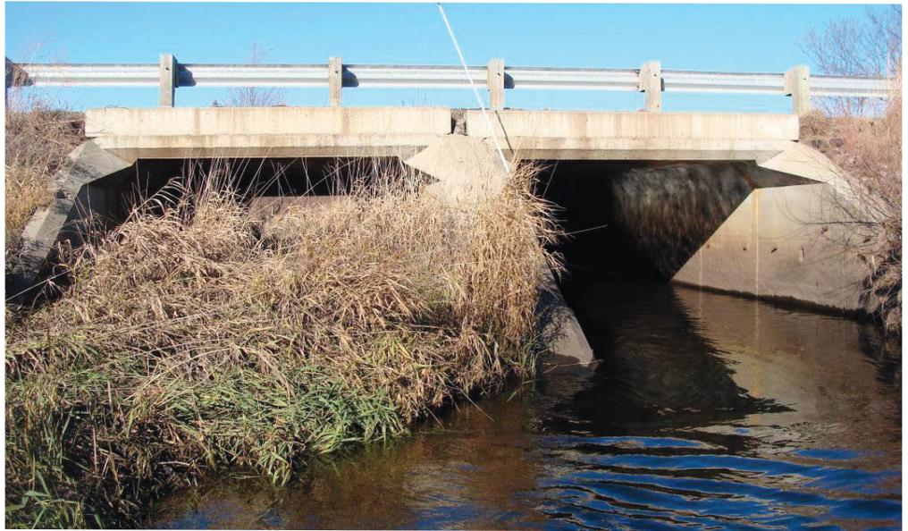
Box culverts are less-expensive alternatives to bridges that allow fish and other aquatic animals to pass under a roadway. When the bottom of the culvert is significantly different from the rest of the stream, however, water flow will also be different, which can make the culvert a barrier to fish passage.
