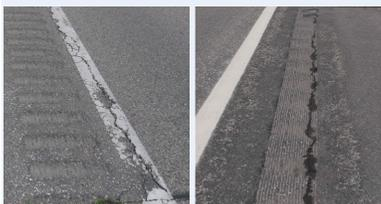
MnDOT's current sharp-edged, rectangular rumble strip design (left) and California's quieter, wave-shaped design (right).
