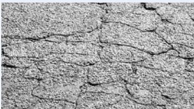
Block cracking indicates that the asphalt binder has oxidized, making the pavement brittle.
