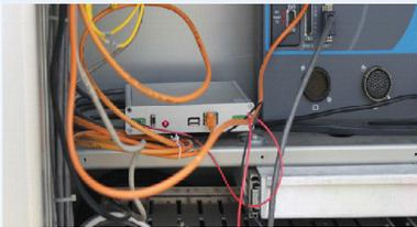
A data collection unit collects event-based traffic and signal data and sends it to a remote center for analysis.
