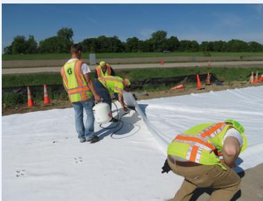
On cells 140 and 240, researchers are comparing geosynthetic layers of different thicknesses for promoting drainage and preventing reflective cracking.
