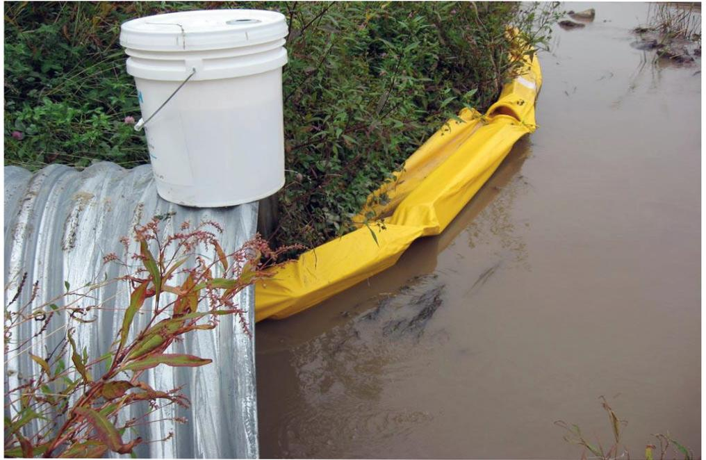
Adding flocculant to stormwater runoff can be as simple as drilling a hole in a bucket of the chemical and mounting it above the water (as shown here), although thorough mixing must be ensured. MnDOT hopes to develop a system that will automatically dispense a precise dose based on the amount of sediment in the water.
