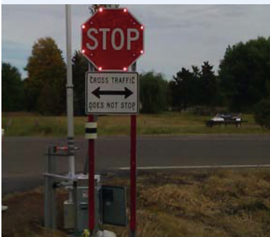
Flashing LEDs make stop signs more conspicuous.
