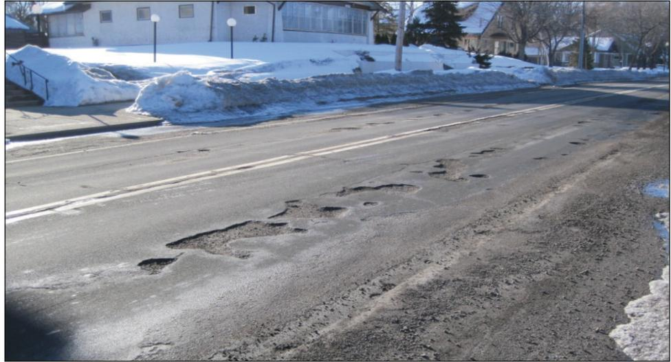
Stripping tends to occur under chip seals of urban curb-and-gutter streets because their closed structure traps water, which can damage asphalt where density is low. Results showed that using a more breathable fog seal instead of a heavier chip seal may help alleviate this problem.
