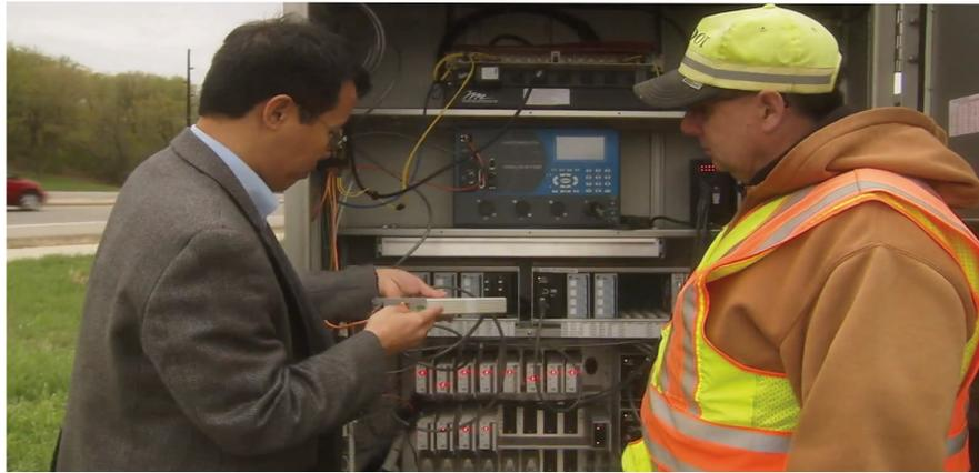
The refined SMART-SIGNAL system's data collection unit is far more compact than its previous iteration and can easily be installed in MnDOT's latest traffic controller cabinets.
