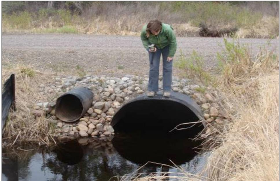
Wide floodplains common in Minnesota sometimes require that culverts be designed with multiple barrels to handle additional flood capacity so that the water velocity in the main barrel does not become too great.
