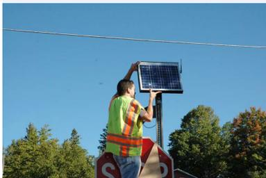
At the test site, solar panels powered the radar detectors mounted at the top of STOP signs located on the secondary road.
