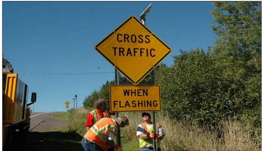
This blinker sign on the main highway is the largest of the three signs installed at the test site. When radar detectors mounted at the top of STOP signs on the secondary road detected vehicles stopped at the STOP signs, a wireless signal transmitted to this sign initiated blinking.
