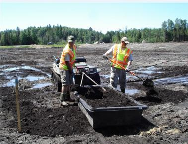
Donor soil was spread by hand over the mitigation site. Because of the wet conditions of the site, soil was hauled using an ARGO amphibious off-road vehicle pulling an Otter sled.
