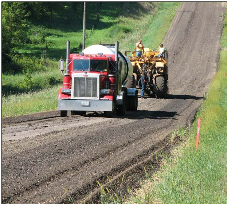
Figure 11. Stabilized Full-Depth Reclamation operation.
