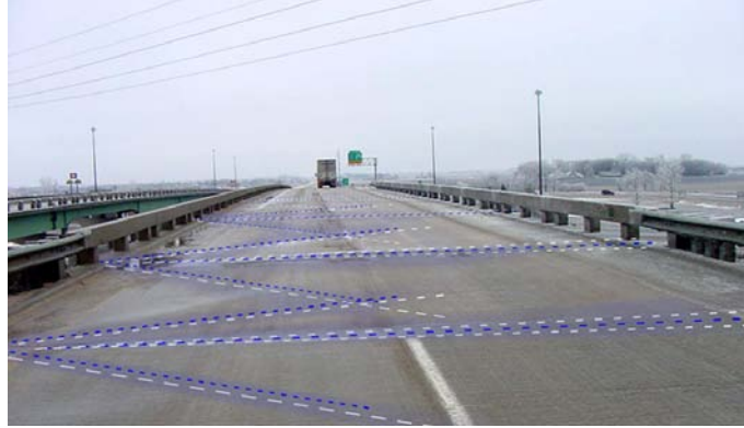
Bridge anti-icing systems help reduce safety issues on bridge decks.
