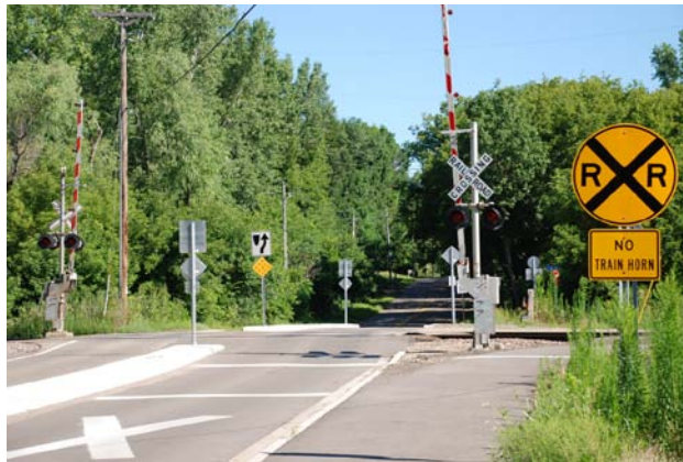
Enhancements are being made to rail crossings to improve safety.
