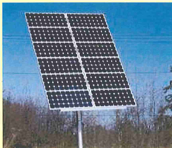
Solar electric panels may also be mounted on a tracking system, which will automatically adjust so that the PV panels face the sun throughout the day.
