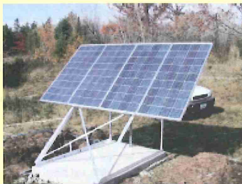
Stationary mounted panels can be adjustable, permitting the panels to face the sun as near to perpendicular as possible.
