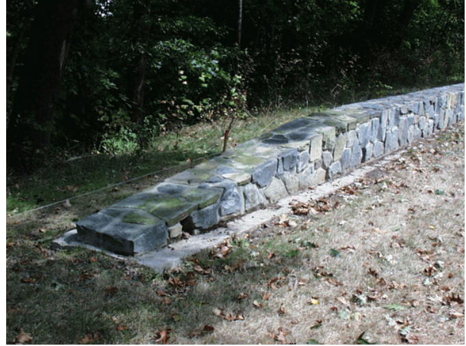
Stone Masonry Guardwall
