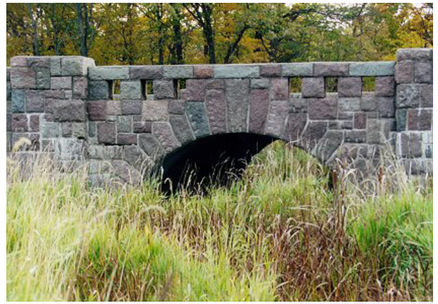
9. East Wall looking West from Lake Edge
