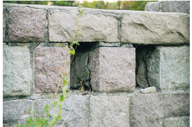
13. Close-up of Joints and Openings in Wall
