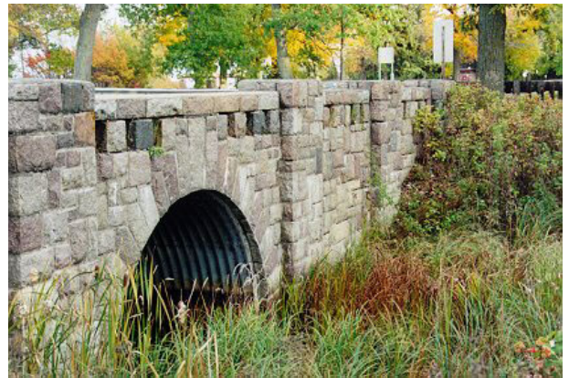
11. North end of West Wall looking Southeast from Median
