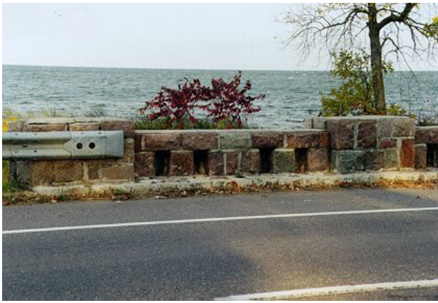
8. North end of East Wall looking East
