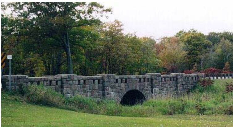
12. East Wall looking Northwest
