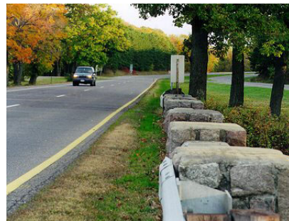
6. West side Wall looking South
