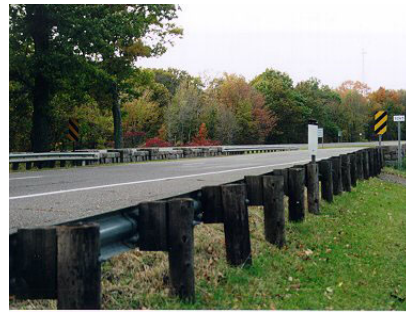
5. East side Guardrail looking North
