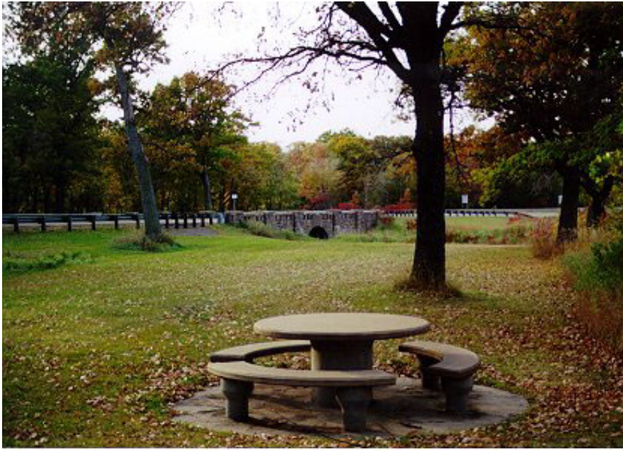
1. View from picnic area looking north at East End of Underpass
