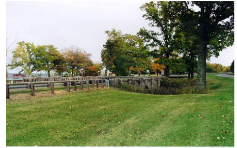
2. Underpass looking South in Median
