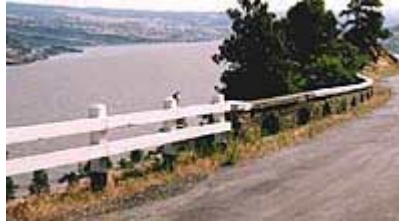
Steel-backed two-rail wooden guardrail
