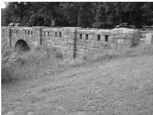
Figure 7. Looking south along the east side of the bridge.
