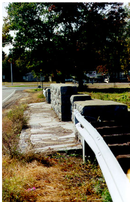
6. West Wall looking South ( overgrown turf )
