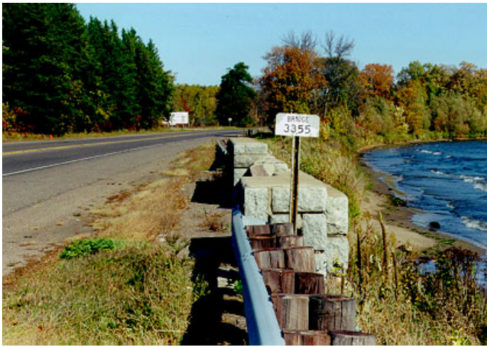
1. East Side looking North
