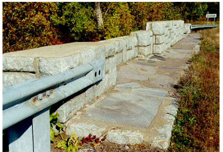
4. West Wall looking North
