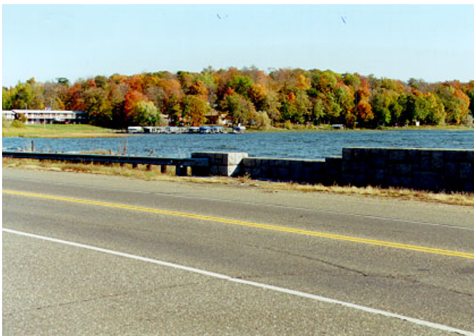
3. North End of the East Wall looking NE
