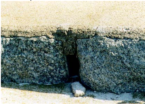
9. Close-up of Mortar Joint Condition.
