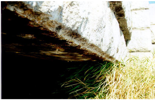
8. Close-up of Granite Header over Culvert
