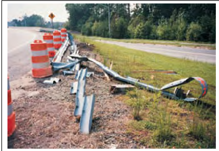
Guardrail Damage
