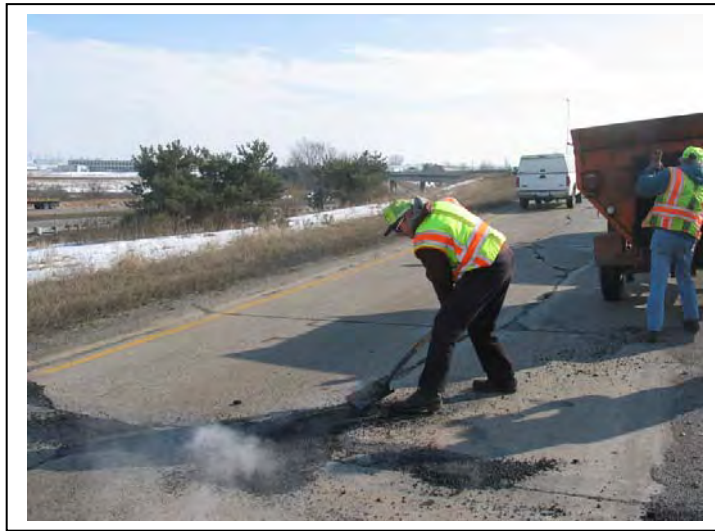
Source: Mn/DOT Office of Maintenance Pavement Patching
