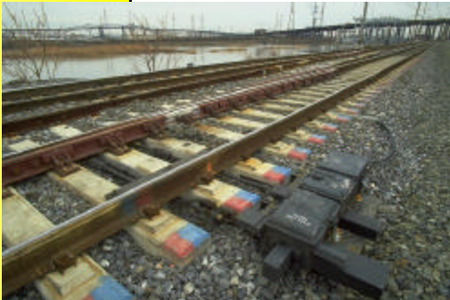
Modern track construction using concrete ties and rail clips.
