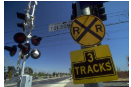
Grade crossing warning equipment and safety are of paramount importance
