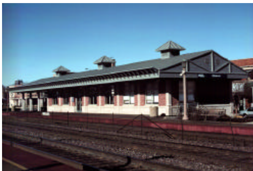
Elmhurst, Illinois Station including Waiting Room, Ticket Sales and Concession
