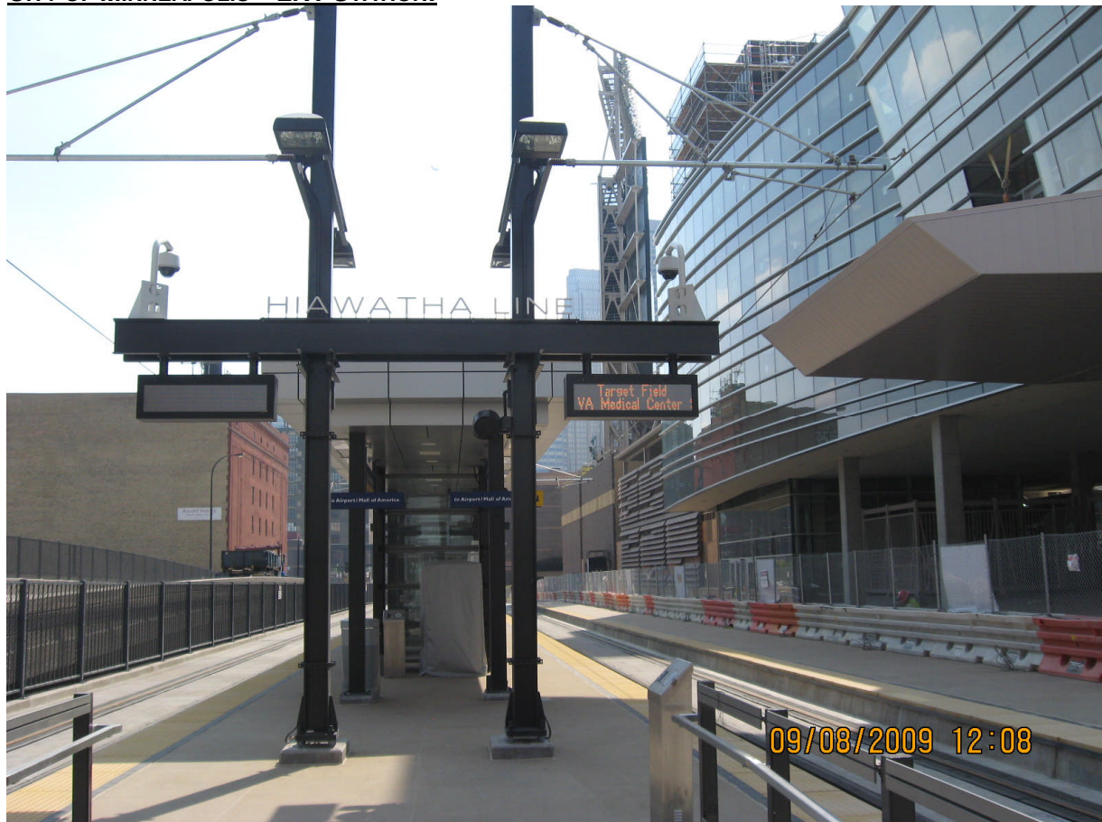
Hiawatha LRT ballpark station (September 8, 2009)
