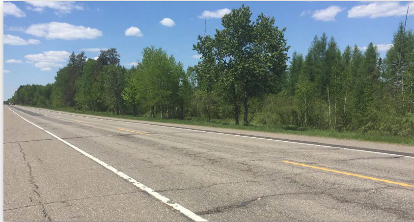
Figure 18: Rough pavement east of Grand Rapids
