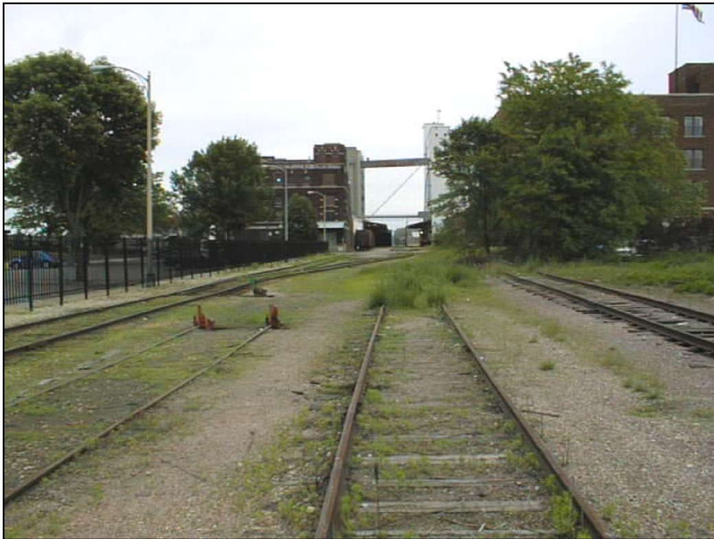
Figure 9-7: Levee Park Yard looking east
