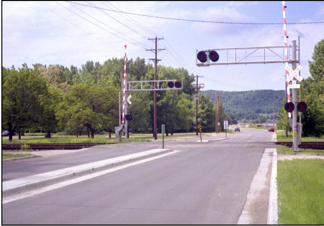
Figure 3-1: Non-mountable center barriers
