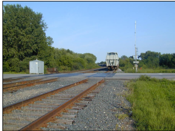
Figure 8-2: Pelzer Street crossing looking east
