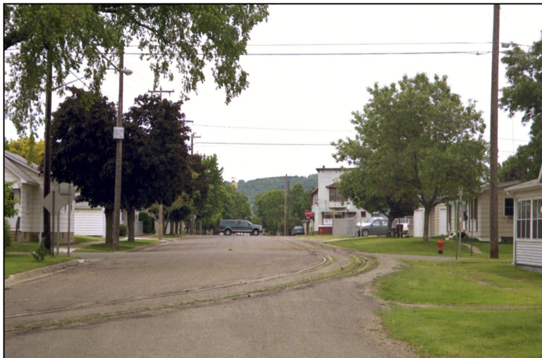
Figure 9-1: CPR Wall Street track is street running (within roadway ROW).
