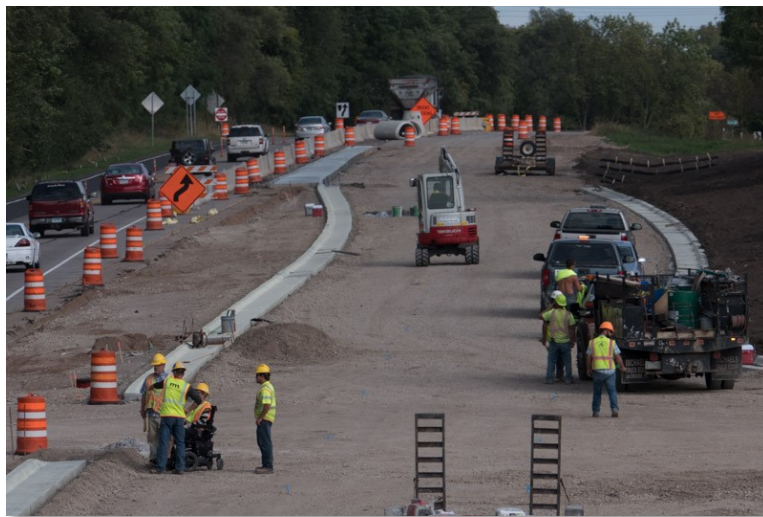
Figure 23: Construction workers rebuild the highway in Red Wing
