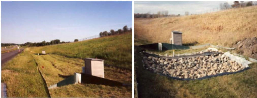
**Figure 3. Vegetative swale (at left) and completed check dam (at right) (from MnDOT 2004-11)**
