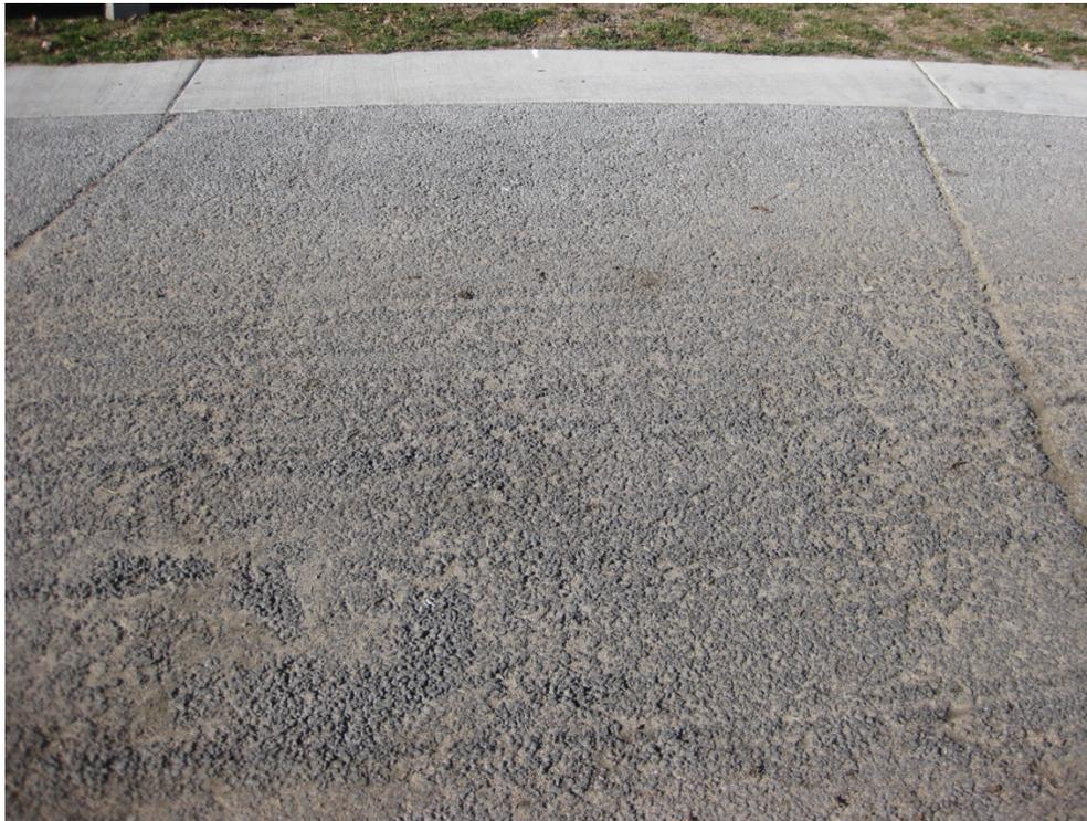
**Figure 7.1 Detroit Lakes Pervious Concrete**
