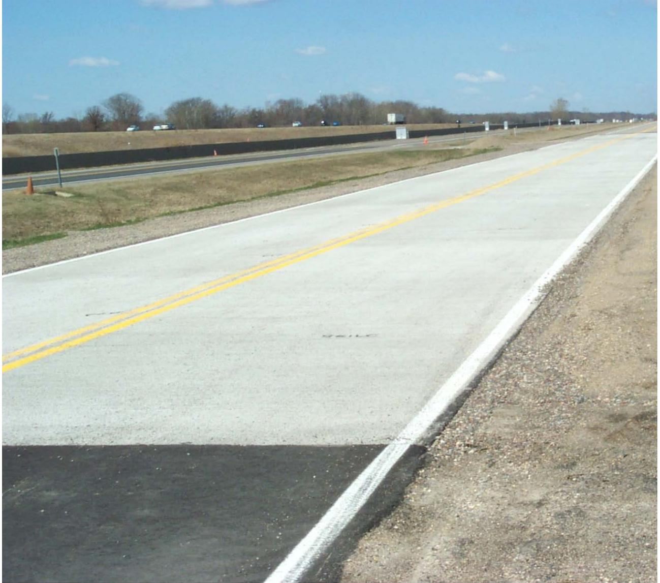
**Figure 3.9: Cell 39 Looking NW Showing Porous Concrete Overlay, Bituminous Transition and French Drain Shouldering Aggregate.**
