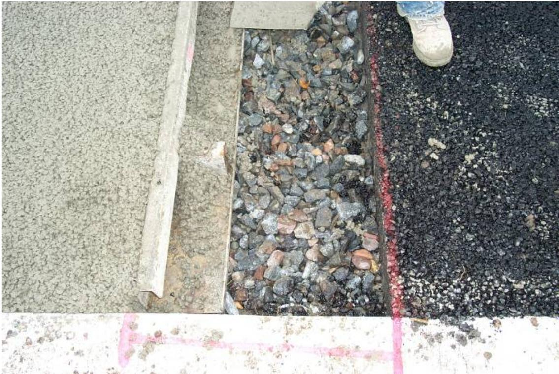
**Figure 3.9: Cell 89 Pervious Concrete on Clay and Cell 88 Porous Asphalt on Clay.**
