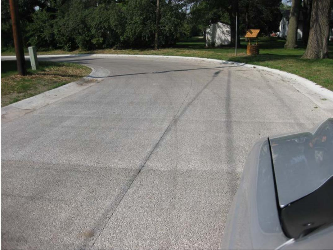
**Figure 7.5 Pervious Concrete in Shoreview**
