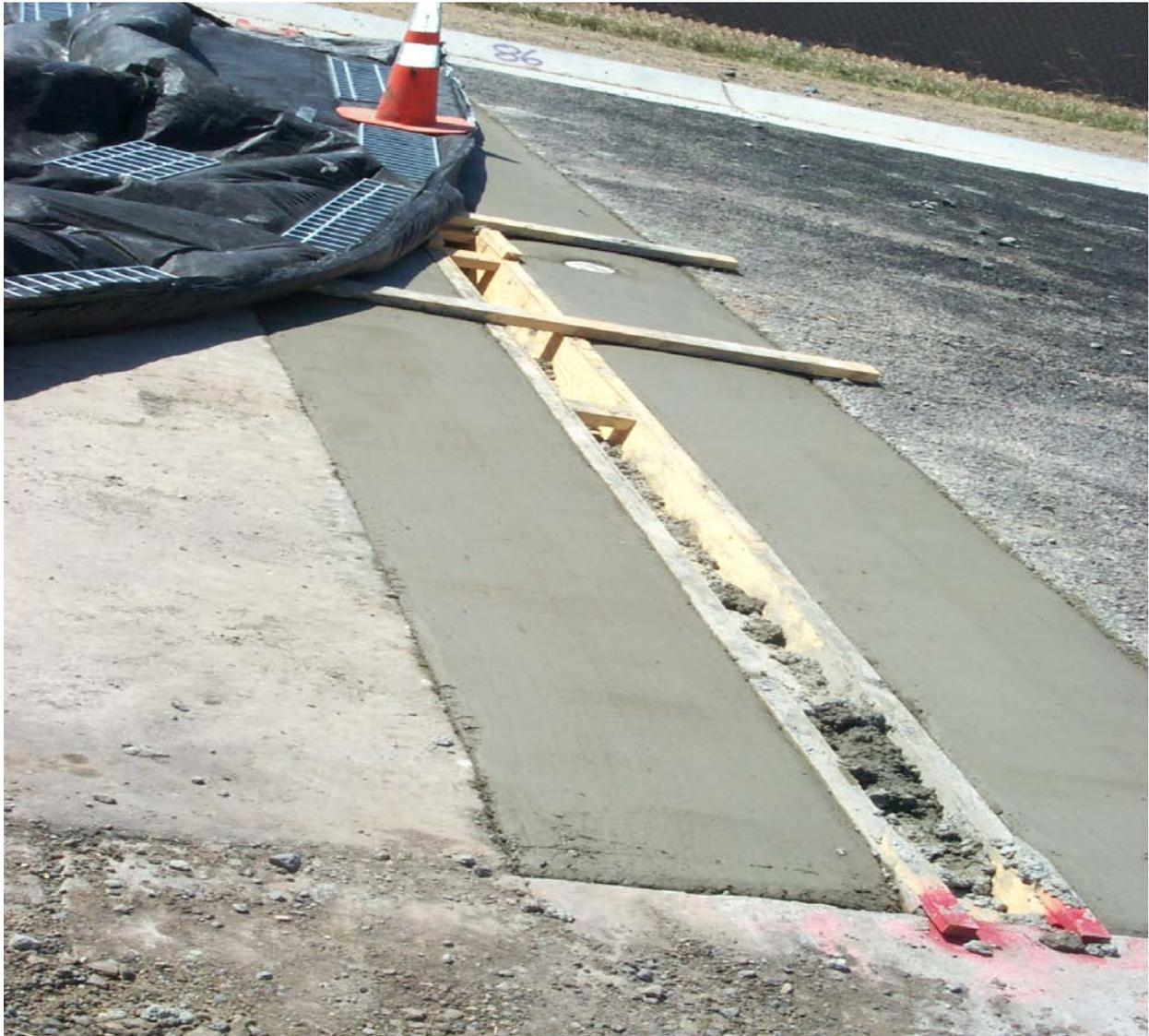
**Figure 3.10: Cross Drain Construction between Porous Cell 86 and Control Cell 87**
