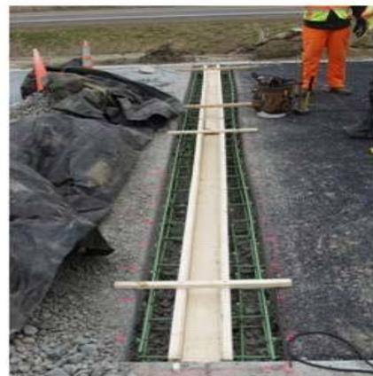
**Figure 5.2: Transverse Drains in Cells 85-89**
