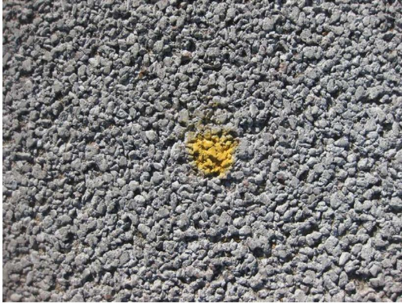
**Figure 7.2 Detroit Lakes Pervious Concrete Surface**
