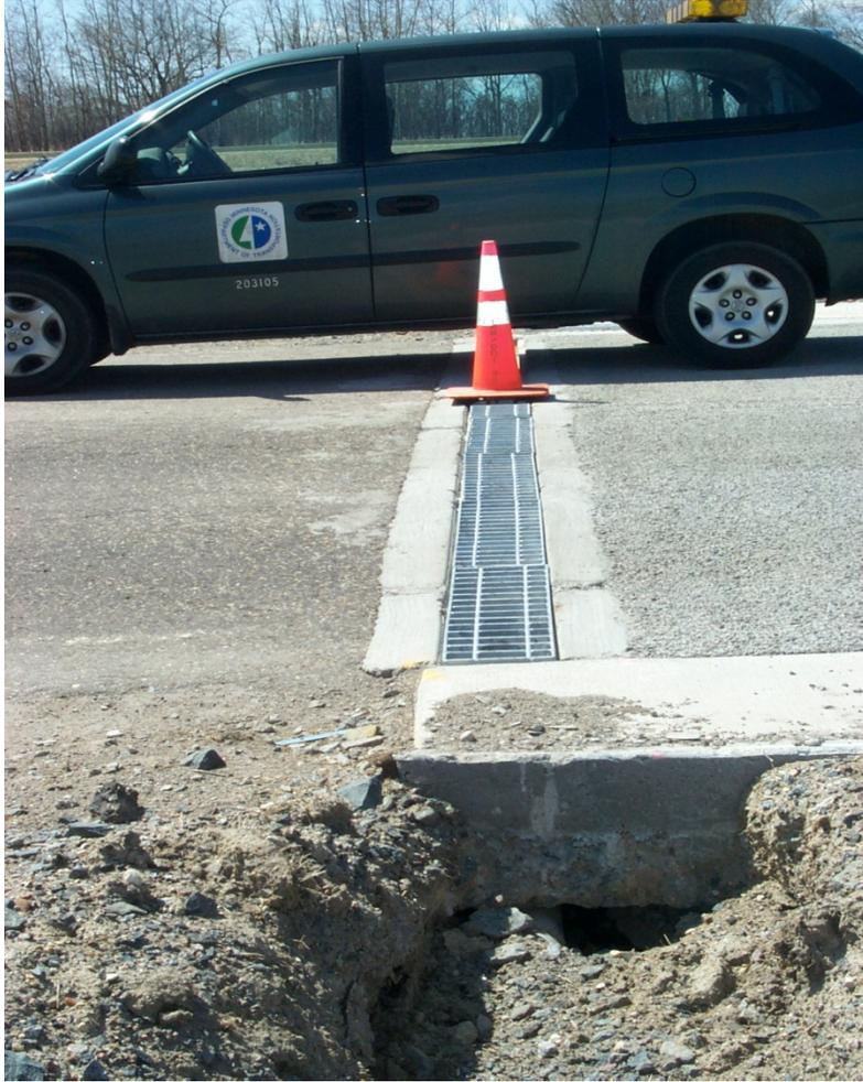
**Figure G2: Covered Cross drains showing Curb and Gutter Boundary**
