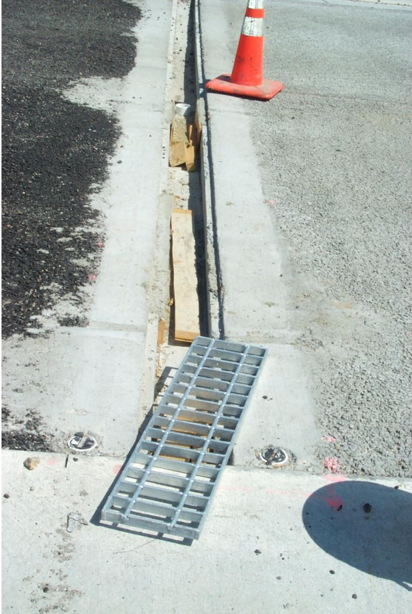
**Figure G3: Cross Drains and Grating**
