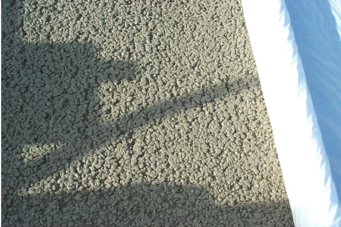
**Figure 3.8: Porous Overlay Surface**
