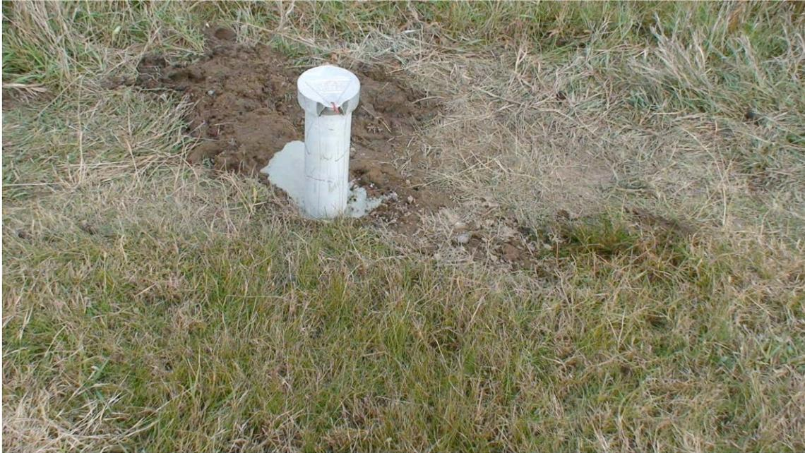
**Figure 2.10: Pervious Well 1 Completed Sand-and-Gravel-Packed, Bentonite-Slurried Cased and Capped.**
