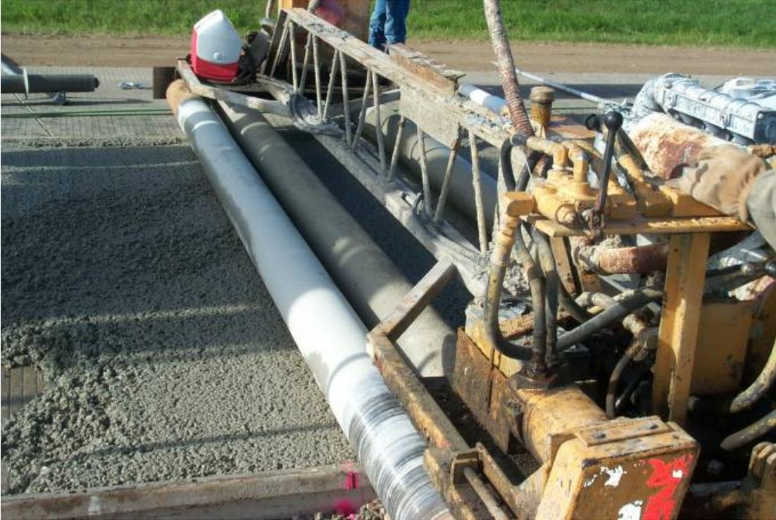
**Figure 3.6: Porous Overlay Compaction**
