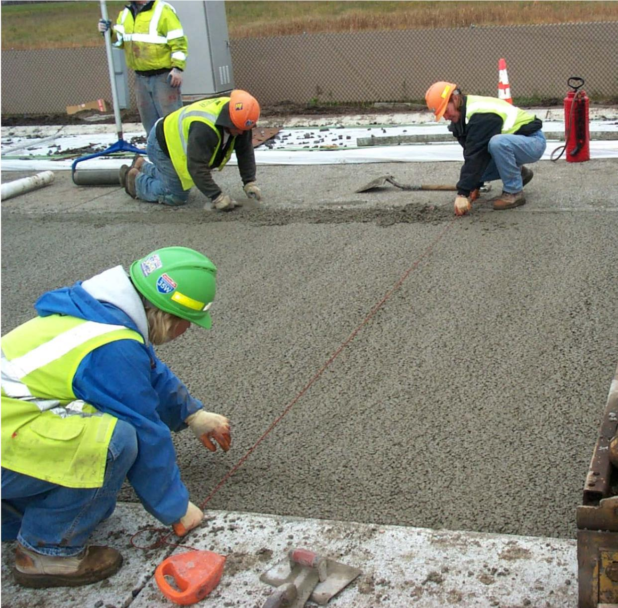
**Figure 3.8: Establishing 10 ft Joints in Cells 85 and 89**
