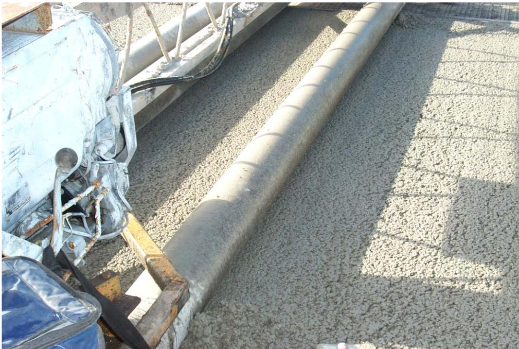
**Figure 3.7: Porous Overlay Multi-Drum Screed Compactor**
