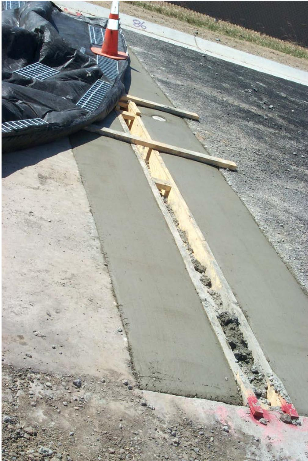
**Figure G7: Cross-Drain Cell 85/Cell 86 Forming and Placement**
