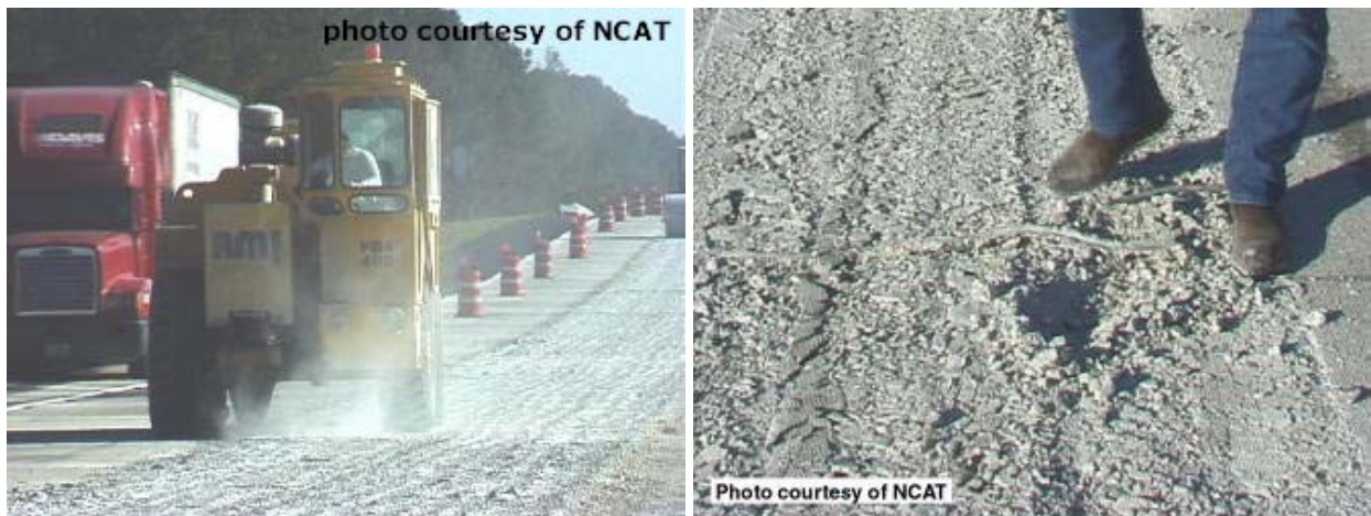
Figure 3.5. At left, resonant pavement breaker used to rubblize PCC pavement; at right, PCC pavement after rubblization with a resonant pavement breaker (WSDOT).
