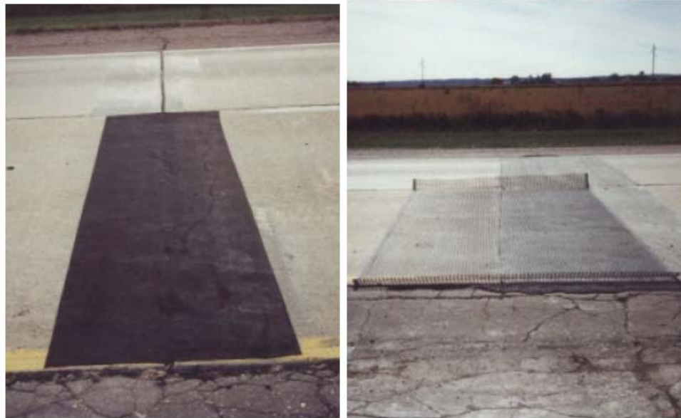
Figure 3.6. Linq-Tac -711N (at left) and Strata Grid-200 geogrid products (Rumpca and Storsten 2000).
