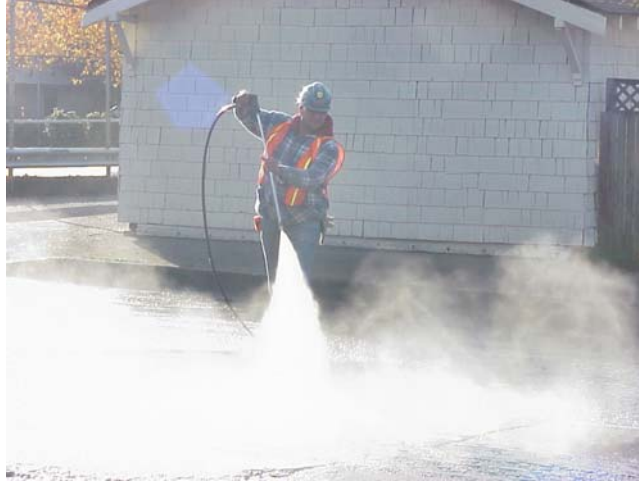
Figure 3.2. Washing the Existing Surface Prior to Overlay (WSDOT).
