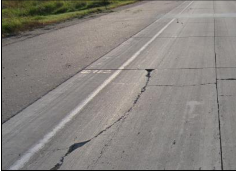
Figure 27: Cracks in Cell 805 in the third year of service.
