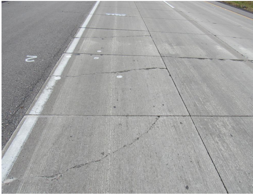
Figure 9: Cracks observed on Cell 506 (replaced in summer 2020).
