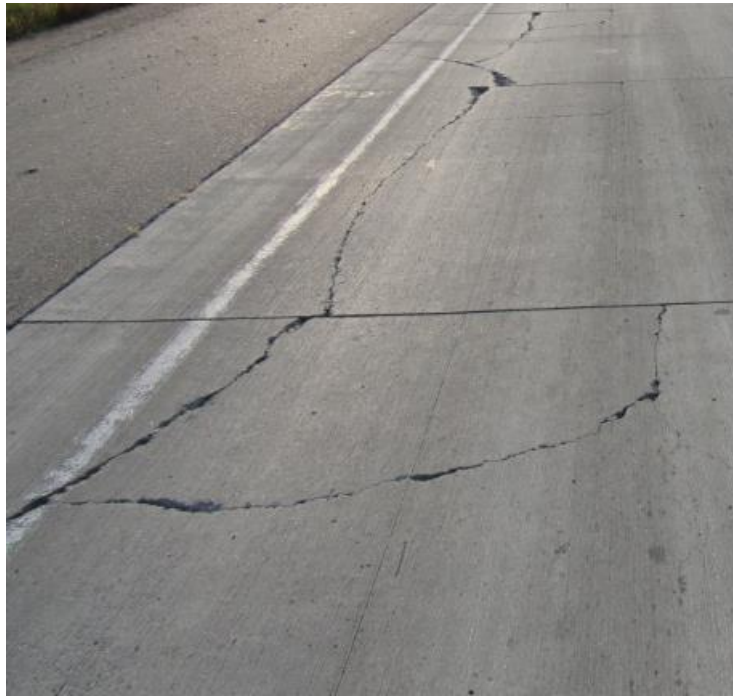
Figure 25: Cracks in Cell 705 in the third year of service.
