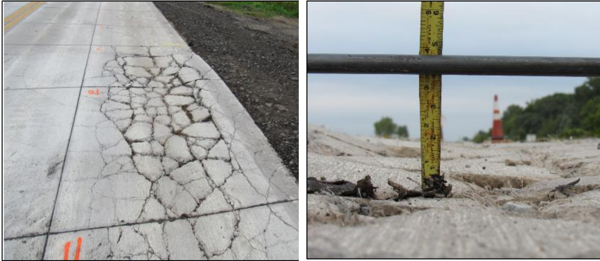
Figure 6: Shattered slabs and depression along the wheel path in Cell 139.
