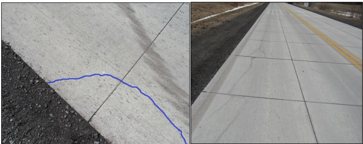
Figure 7: Corner and longitudinal cracks in Cell 239.
