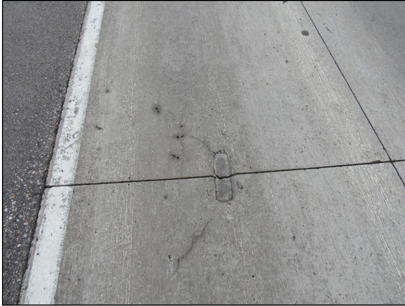
Figure 3-15. Narrow cracks in Cell 806, originated at the location of the joint opening sensor
