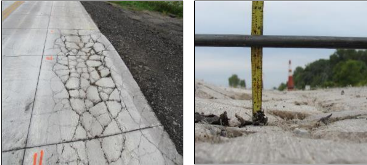
Figure 3-2: Shattered slabs and depression along the wheel path in Cell 139 after MnROAD truck loadings.
