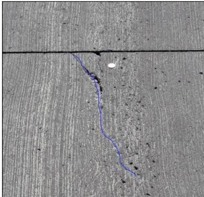
Figure 3-22. Longitudinal crack in Cell 805 (2018)
