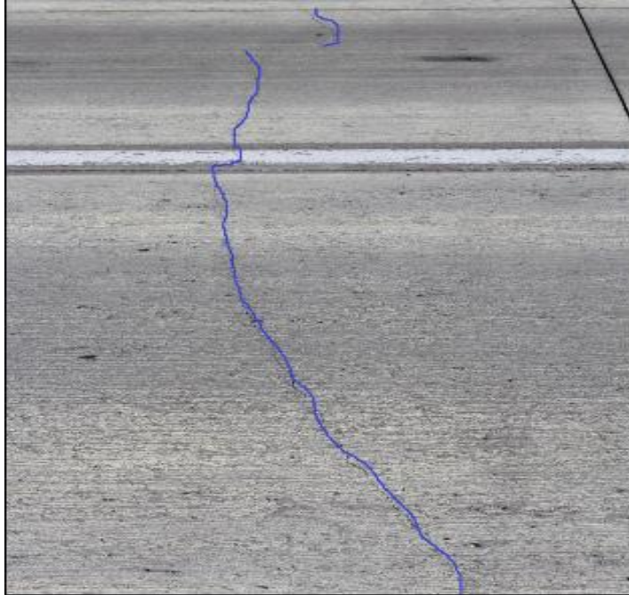
Figure 3-23. Transverse crack in Cell 805 (2018)
