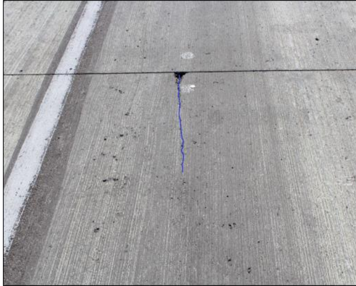
Figure 3-17. Longitudinal crack in Cell 705 (2018).
