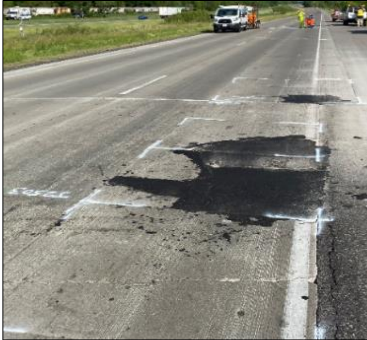
Figure 3-11. Cell 506 before replacement on June 2020
