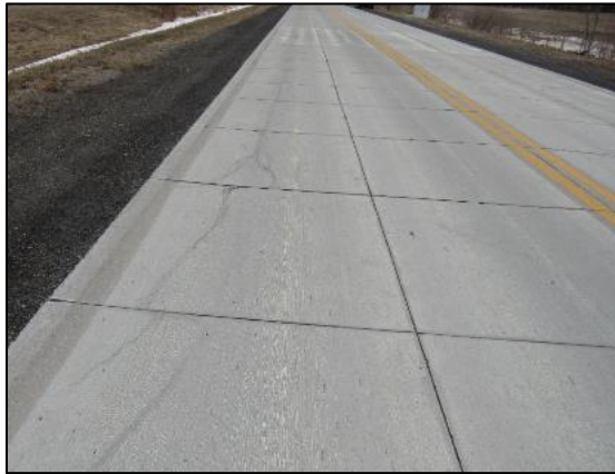
Figure 3-6. Longitudinal cracks in Cell 239 (April 2019)
