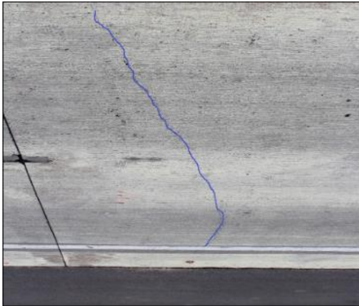
Figure 3-18. Transverse crack in Cell 705 (2018).
