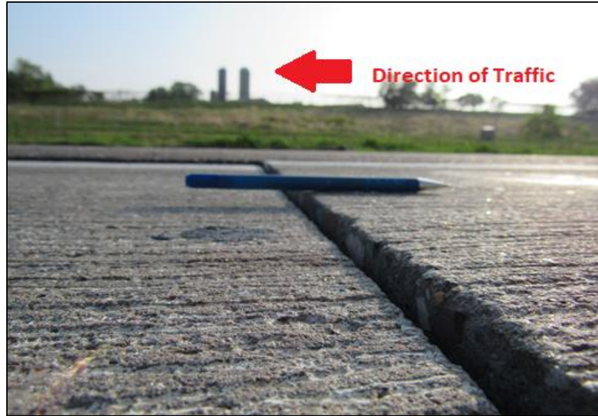
Figure 4-3. Photograph of faulting of Cell 506 (non-FRC). Note that faulting is exaggerated due to the broken corner in the slab on leave slab.
