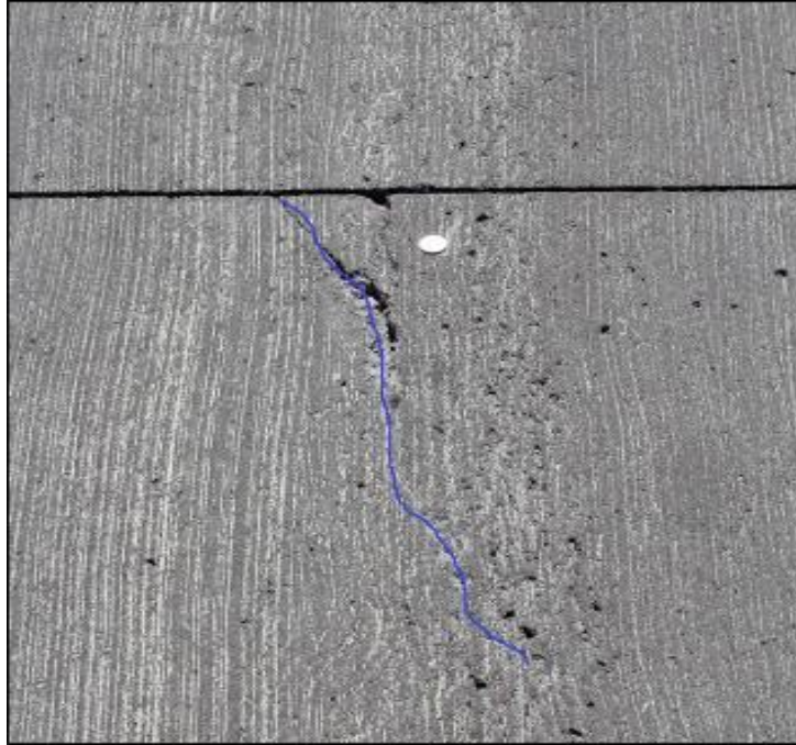
Figure 2-15. Longitudinal crack in Cell 805 (2018)
