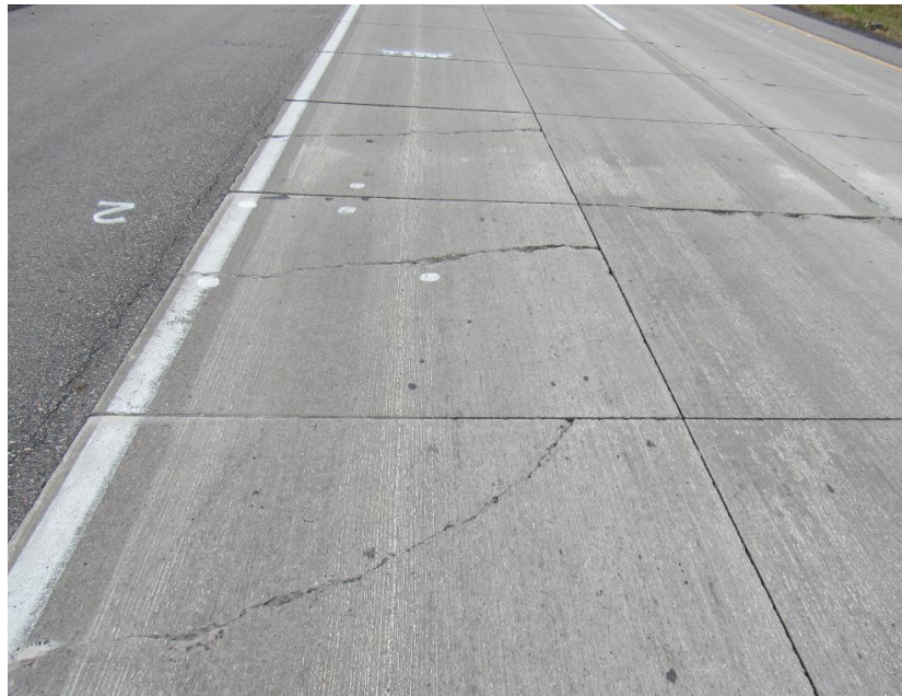
Figure 2-22. Photographs of transverse and diagonal cracks in Cell 506 (October 2019)
