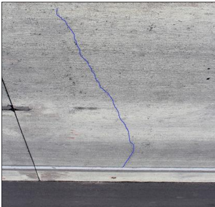
Figure 2-11. Transverse crack in Cell 705 (2018)
