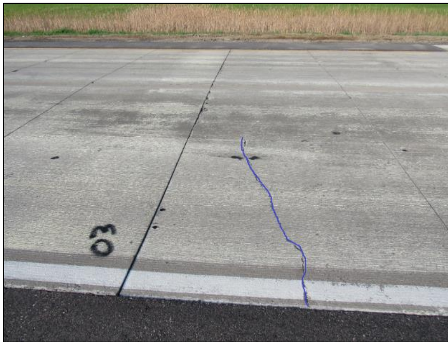
Figure 2-20. Transverse crack in Cell 506 (control, non-FRC) observed in the year 2018.
