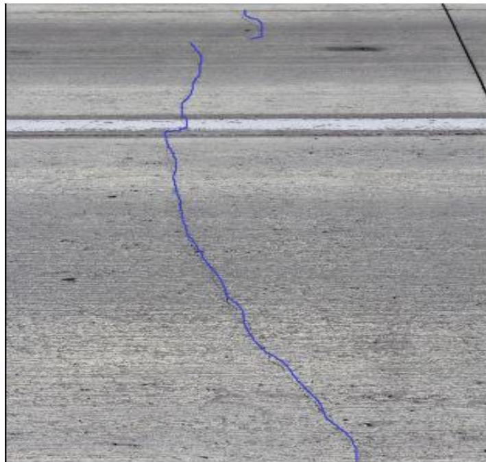
Figure 2-16. Transverse crack in Cell 805 (2018)
