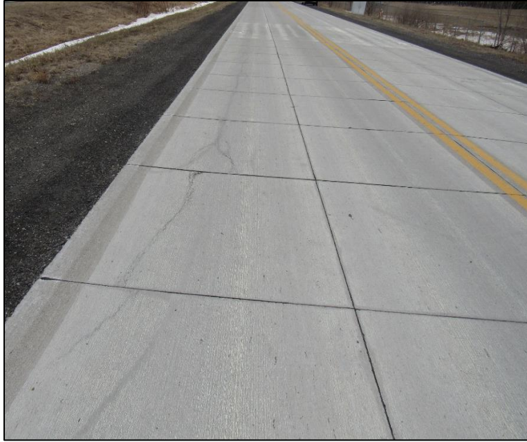
Figure 2-9. Longitudinal cracks in Cell 239 (April 2019)
