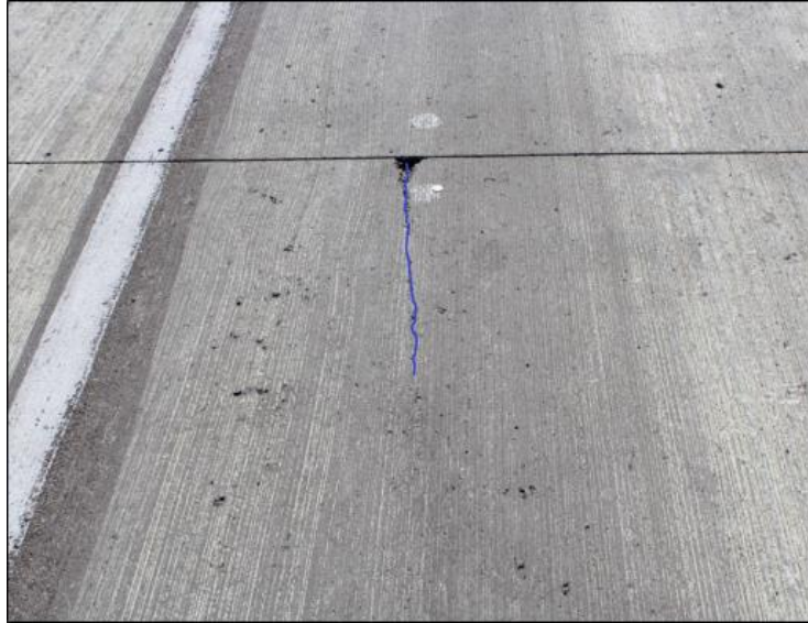
Figure 2-10. Longitudinal crack in Cell 705 (2018)
