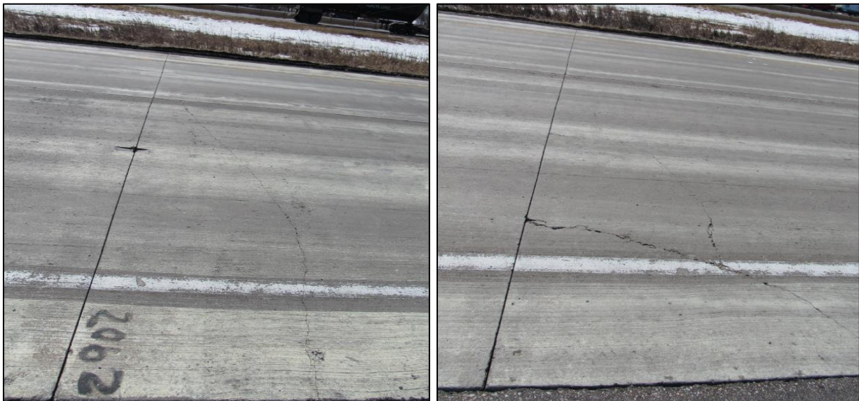
Figure 2-13. Photographs of transverse and corner cracks in Cell 705 as observed during April 2019
