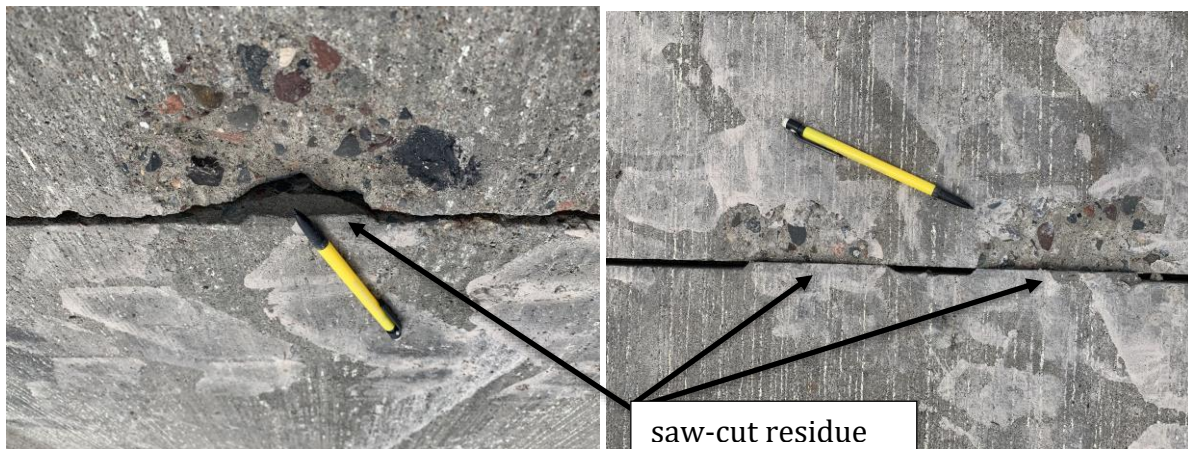
Figure 2-24. Hardened saw-cut residue found within the spalled joints of Cell 506.
