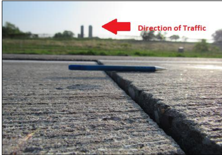
Figure 2-30. Photograph of faulting of Cell 506 (non-FRC). Note that faulting is exaggerated due to the broken corner in leave slab.
