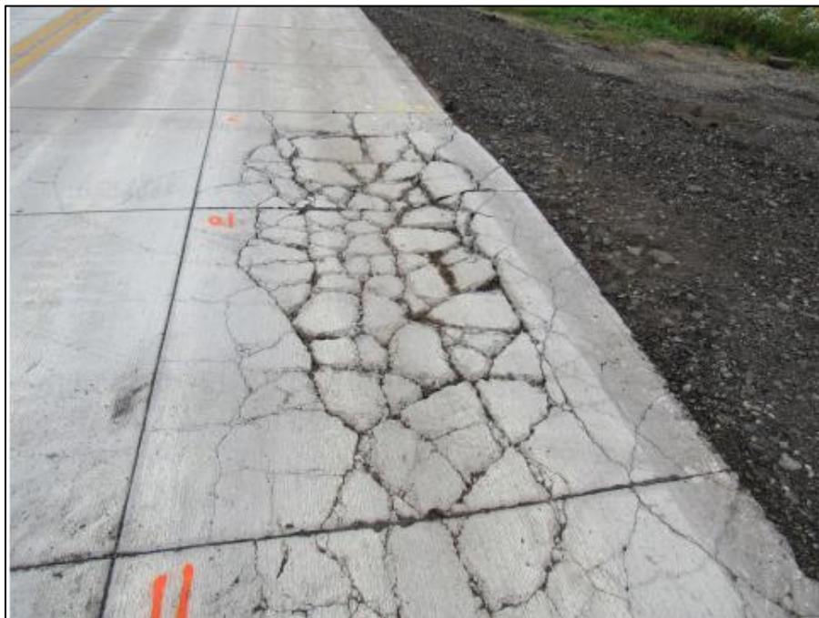
Figure 2-3. Shattered slabs in Cell 139 .
