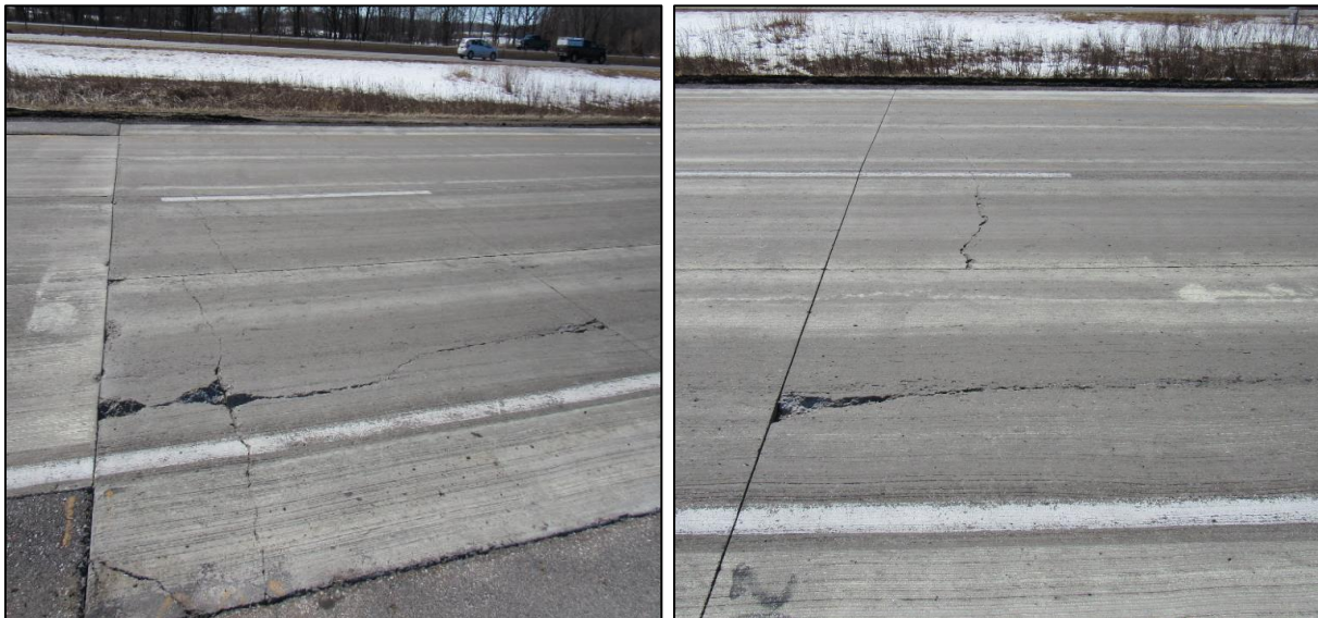
Figure 2-18. Photographs of observed cracks in Cell 805 during April 2019.
