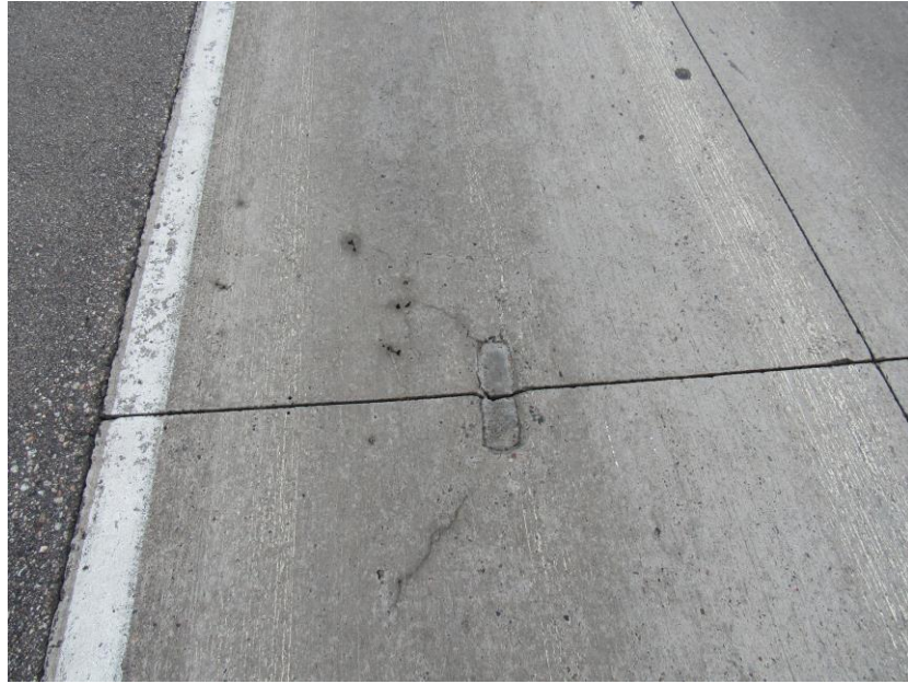
Figure 2-26. Narrow cracks in Cell 806, originated at the location of the joint opening sensor
