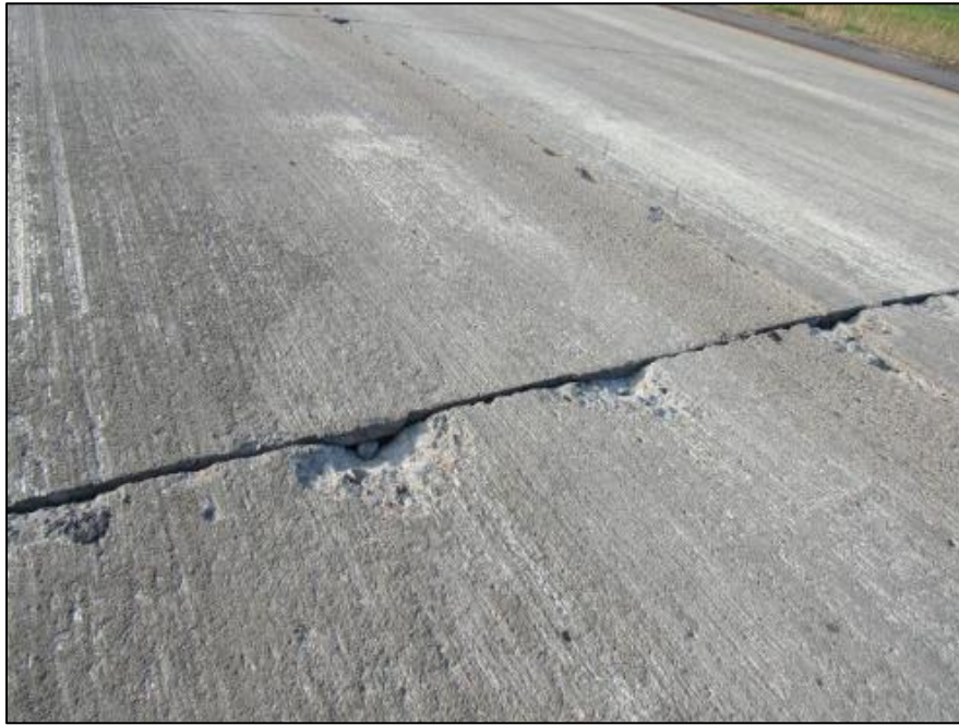
Figure 2-21. Spalling in Cell 506 (control, non-FRC) observed in the year 2018.
