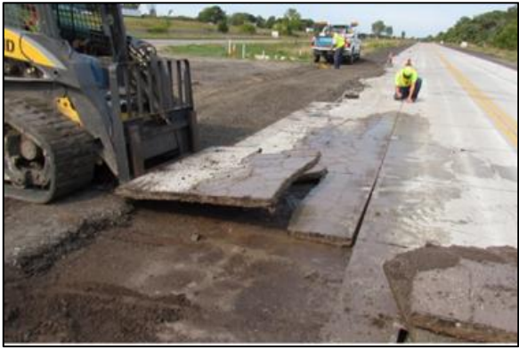
(2.5 a) Removal of broken slabs for Cell 139
