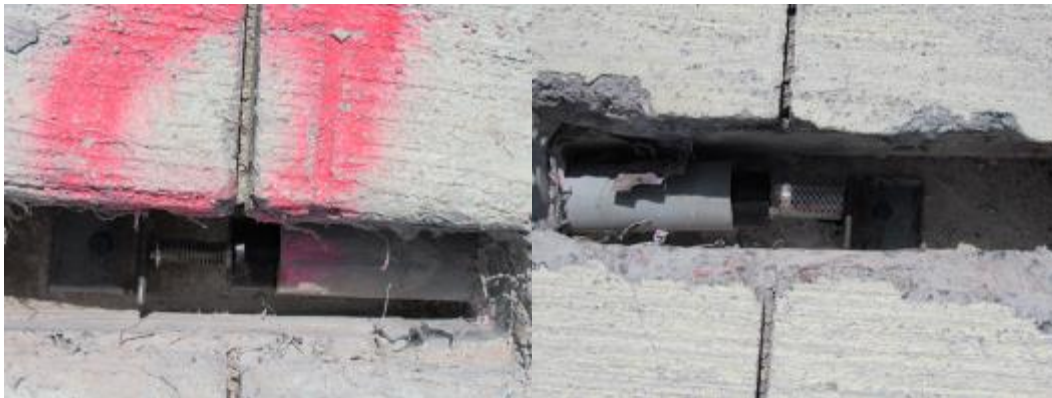
Figure 3-39. Sketch and photographs of joint opening sensors before installation of protective covering.
