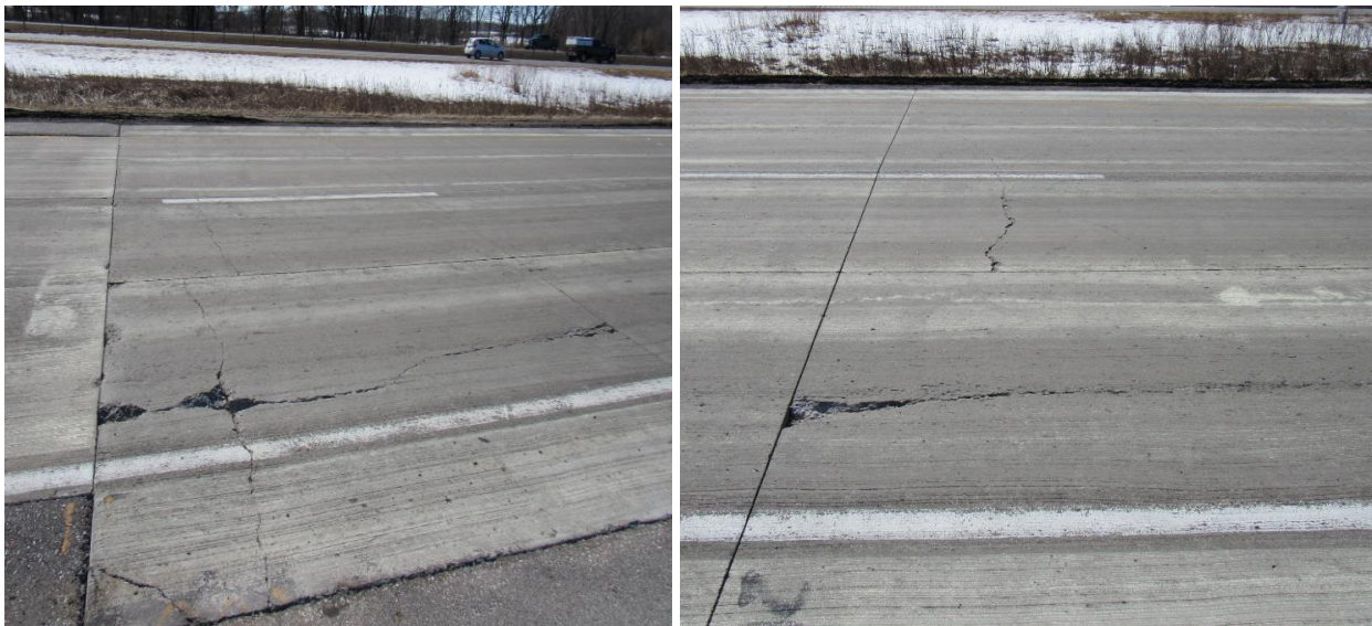
Figure 2-17. Photographs of observed cracks in Cell 805 during April 2019.
