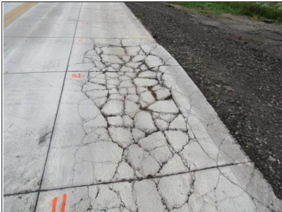
Figure 2-3. Shattered slabs in Cell 139 .
