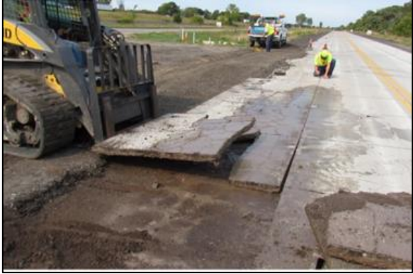
(2.5 a) Removal of broken slabs for Cell 139
