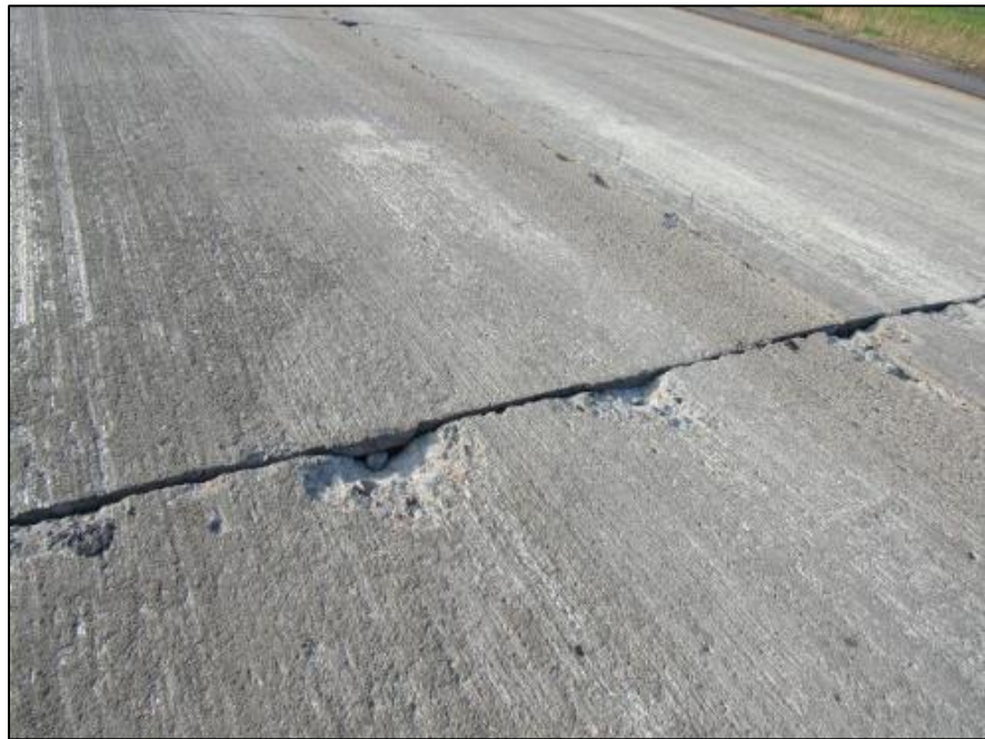
Figure 2-19. Spalling in Cell 506 (control, non-FRC) observed in the year 2018.
