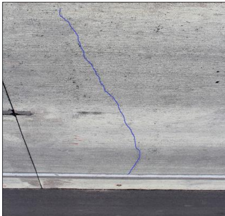
Figure 2-11. Transverse crack in Cell 705 (2018)
