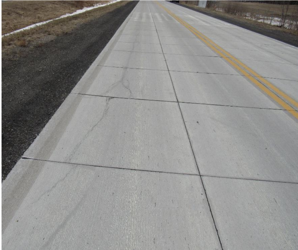
Figure 2-9. Longitudinal cracks in Cell 239 (April 2019)
