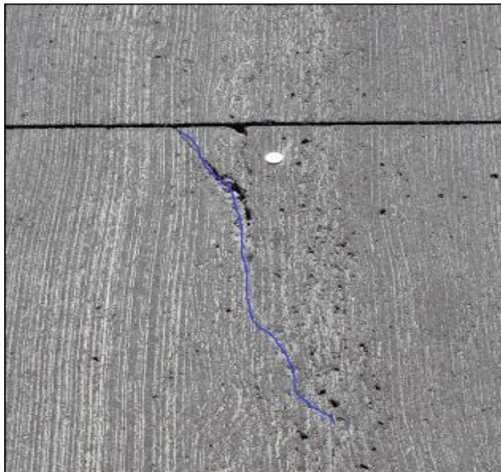
Figure 2-13. Longitudinal crack in Cell 805 (2018)
