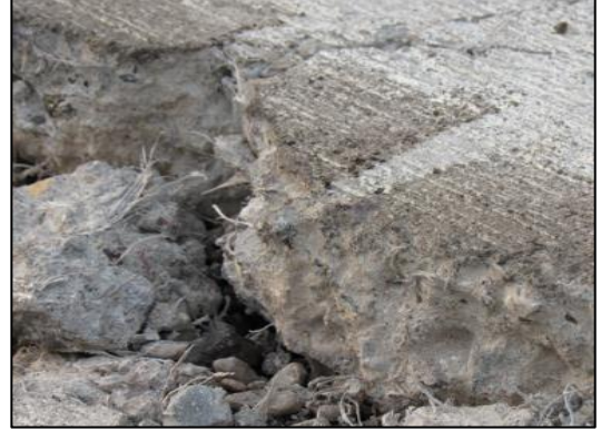
(2.5b) Close shot of the broken concrete pieces
