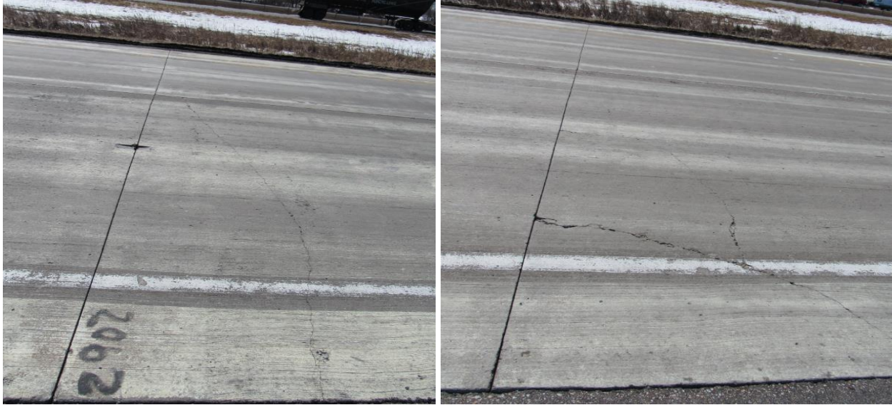
Figure 2-16. Photographs of transverse and corner cracks in Cell 705 as observed during April 2019
