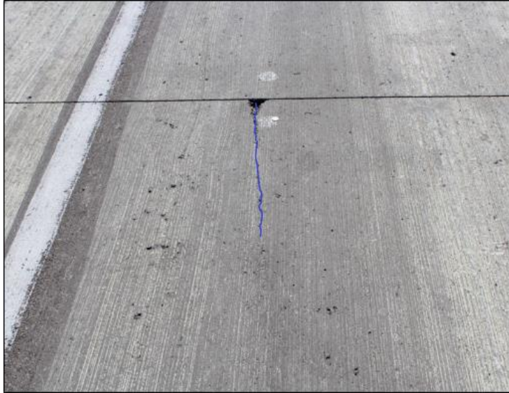
Figure 2-10. Longitudinal crack in Cell 705 (2018)
