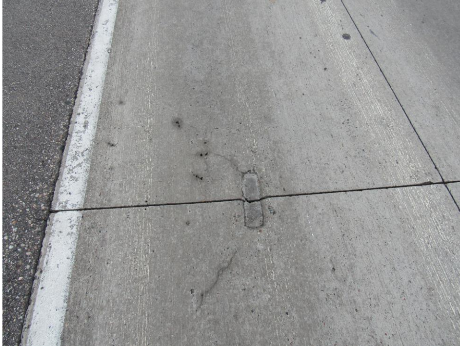
Figure 2-22. Narrow cracks in Cell 806, originated at the location of the joint opening sensor
