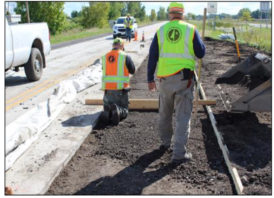
(2.5d) Preparation of the base layer for reconstruction of the broken slabs.
