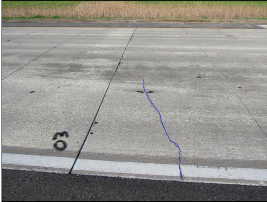
Figure 2-18. Transverse crack in Cell 506 (control, non-FRC) observed in the year 2018.
