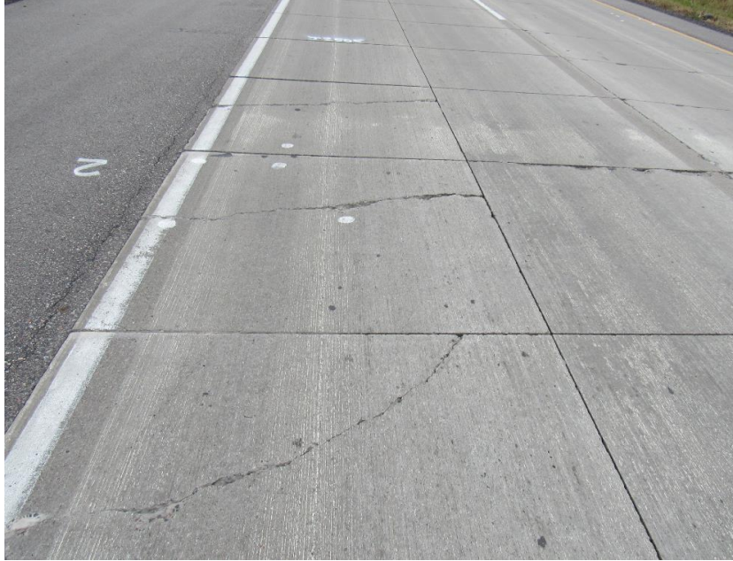
Figure 2-20. Photographs of transverse and diagonal cracks in Cell 506 (October 2019)
