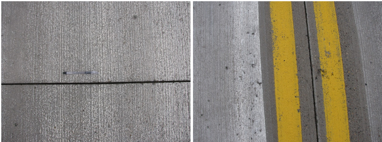
Figure 13- Typical surface quality at cell 138 (left), and finishing issues observed at cell 238 (right)
