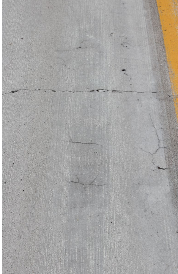
Figure 12- Distress in form of map cracking near the wheel path at cell 238
