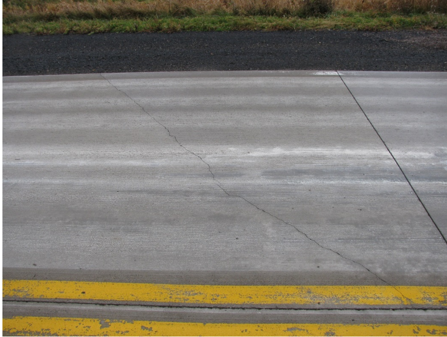
Figure 11- Cracking occurred on inside lane at cell 138
