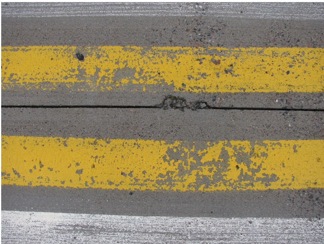
Figure 22- Typical condition of longitudinal joints (top) and occasional raveling (bot.) at cell 138
