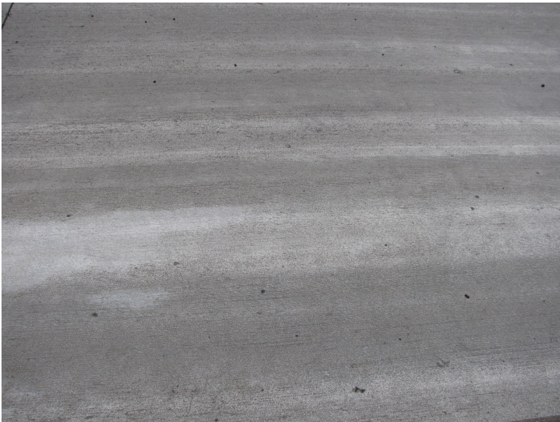
Figure 21- Examples of typical pavement surfaces at cell 138
