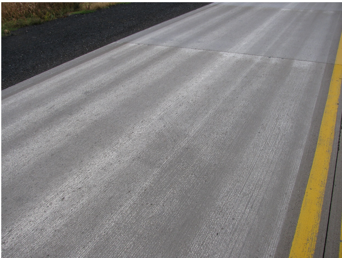
Figure 20- Examples of typical pavement surfaces at cell 238, outside lane (top), inside lane (bot.)
