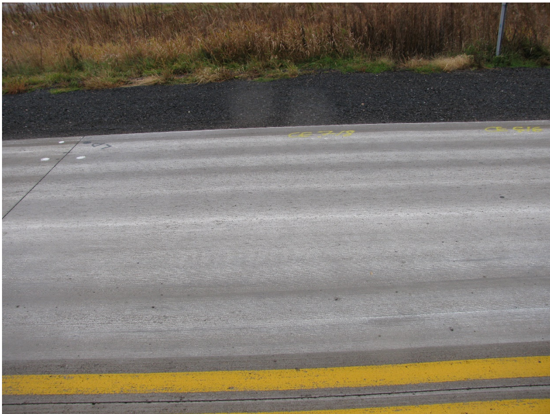
Figure 17- Examples of typical pavement surfaces at cell 138
