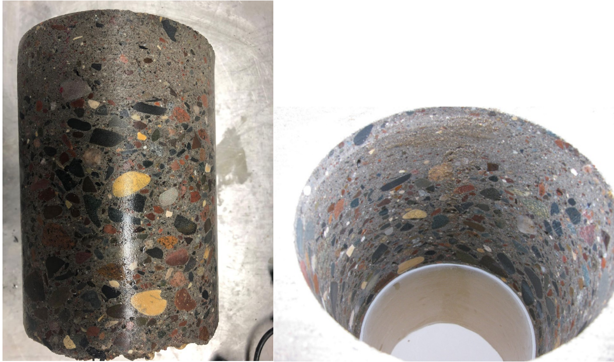
Figure 28- Segregation of coarse aggregate in distress area; Core T-1 (Left) and corresponding core hole (Right)
