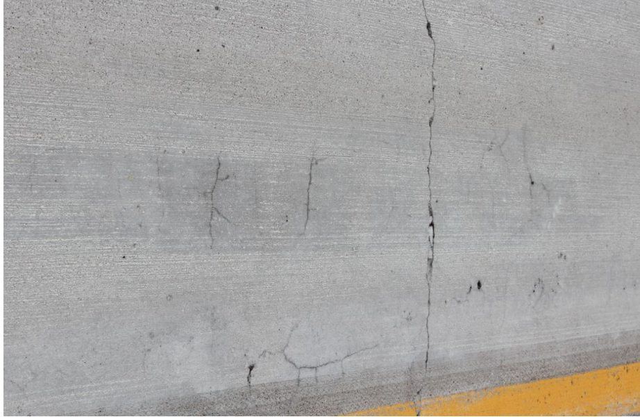
Figure 32- Further distress in form of cracking near the wheel path at Cell 238
