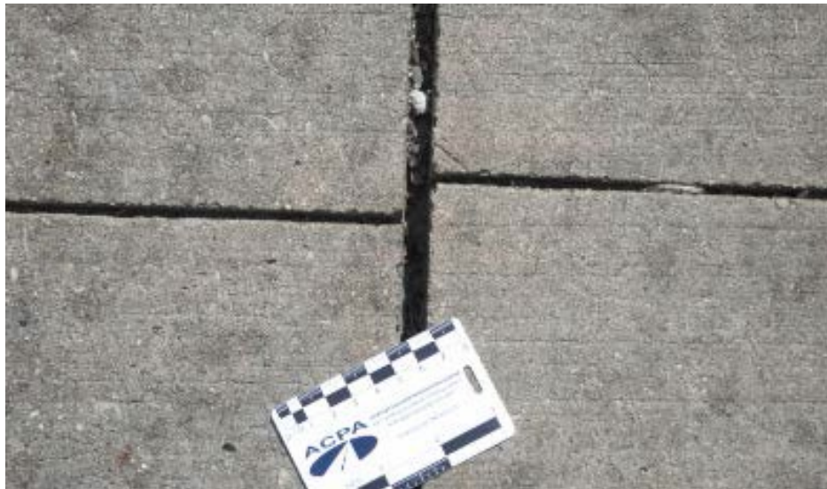
Figure 4-2. Slab migration at the outside longitudinal joint of a overlay project in Illinois (Schank Avenue, Mundelein: (King and Roesler, 2014))
