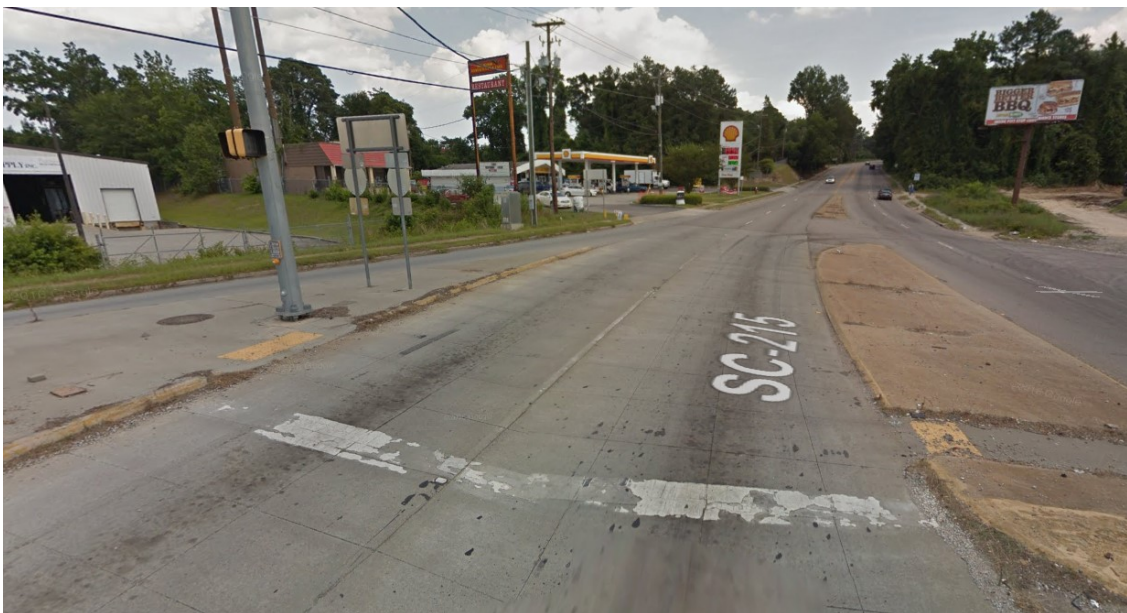
Figure 4-7. Whitetopping project on SC-215 near Columbia, SC (Google Maps, 2016)
