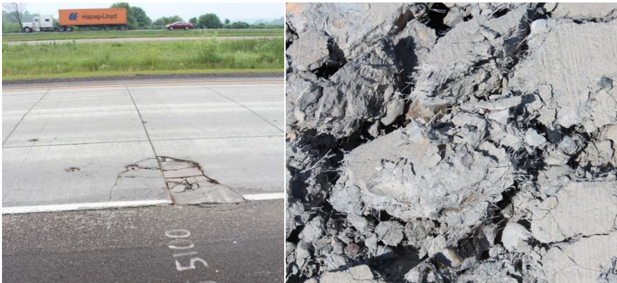
Figure 4-5. (a) Localized distress in Cell 162, (b) concrete broken to replace the slab (Burnham and Andersen, 2015)
