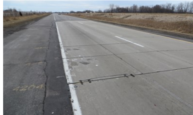
Joint faulting
