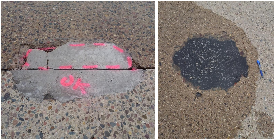
Figure 5.24 Cell 94008 (A) – General condition, missing/replaced material (Rating – 0)
