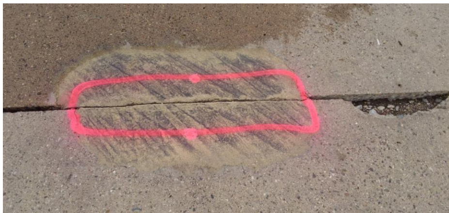
Figure 5.12 Cell 94004 (A) – General condition, debonding (Rating – 3)
