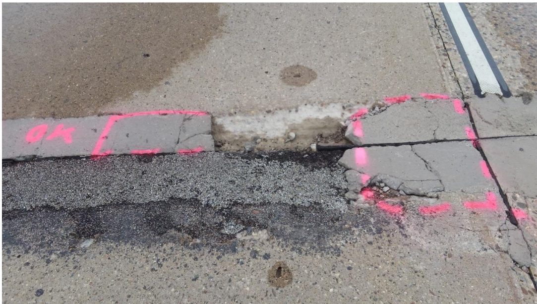
Figure 5.26 Cell 94008 (B) – General condition, cracks and missing material (Rating – 1)
