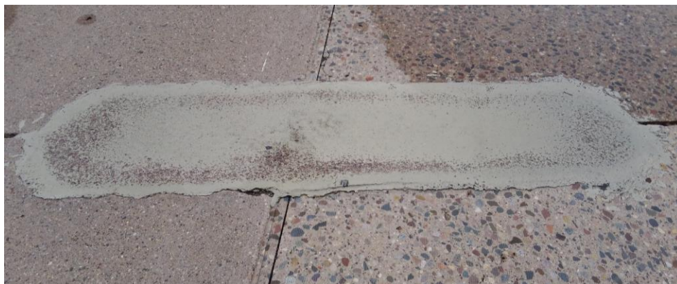
Figure 5.30 Cell 94010 – General condition, no distress (Rating – 4)
