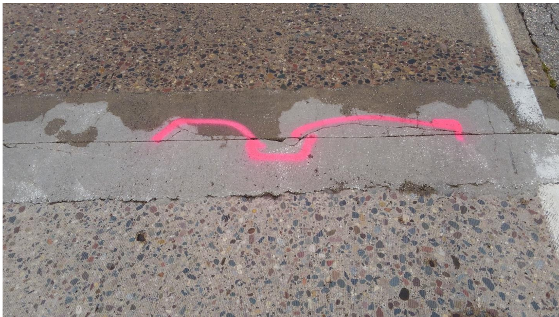
Figure 5.8 Cell 94003 (A) – General condition, linear cracks and debonding (Rating – 3)
