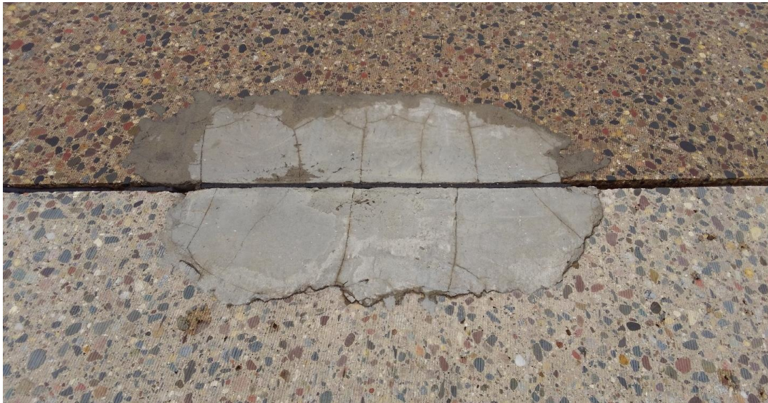
Figure 5.4 Cell 94002 (A) – General condition, linear cracks (Rating – 3)
