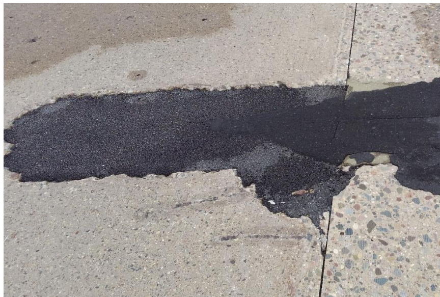
Figure 5.20 Cell 94006 (B) – General condition, over 50% repaired (Rating – 1)
