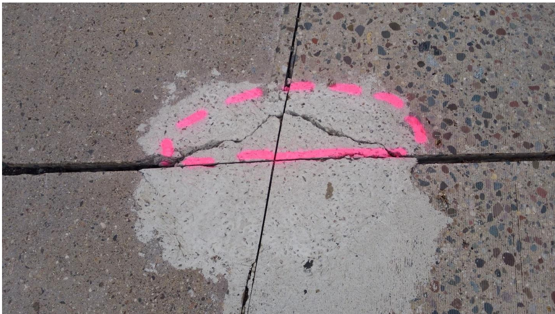
Figure 5.38 Cell 94013 (B) – General condition, cracking and debonding (Rating – 3)
