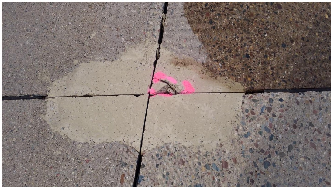
Figure 5.34 Cell 94012 – General condition, cracking and debonding (Rating – 3)
