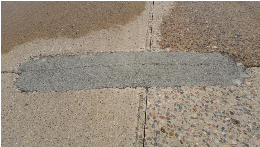
Figure 5.14 Cell 94004 (B) – General condition, linear cracks (Rating – 3)
