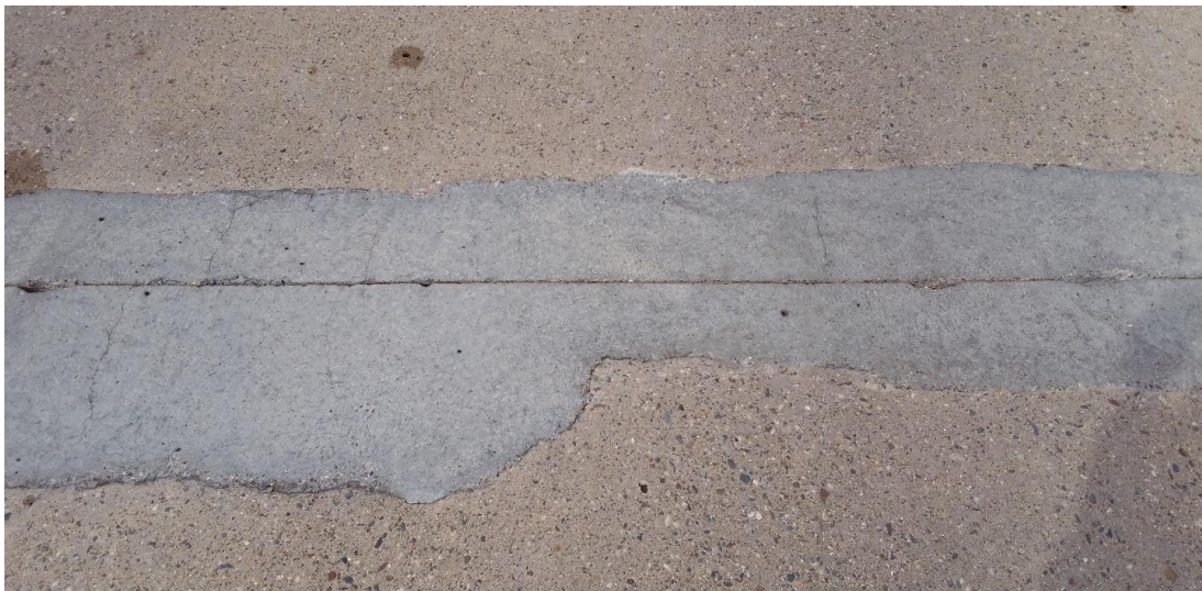
Figure 5.32 Cell 94011 – General condition, no distress (Rating – 4)
