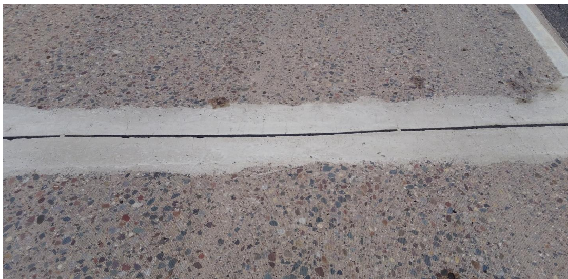
Figure 5.2 Cell 94001 – General condition, minor shrinkage cracks (Rating – 4)
