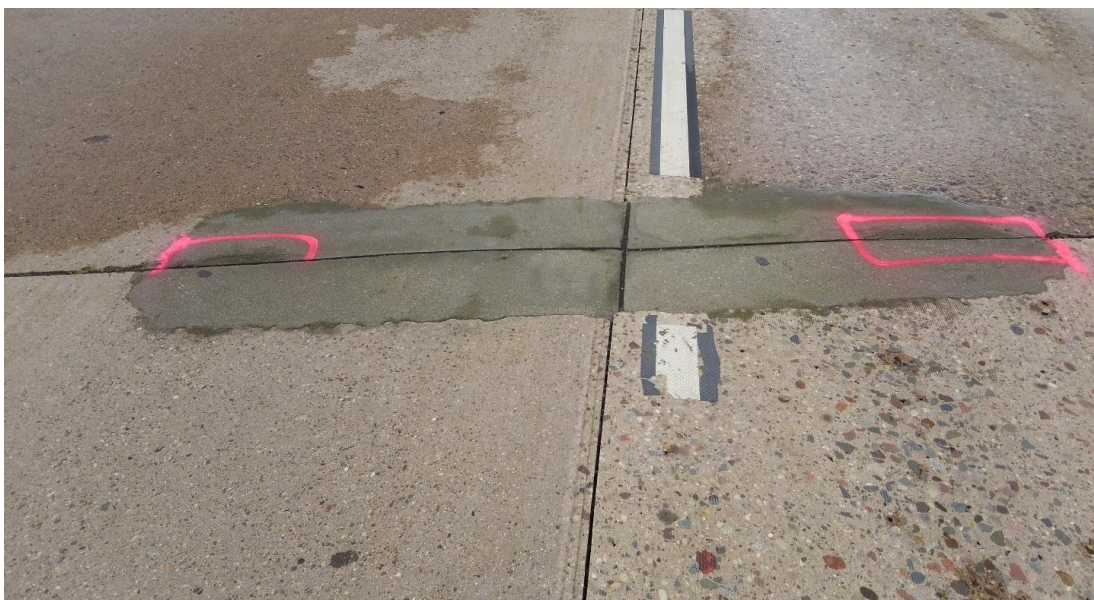
Figure 5.16 Cell 94005 – General condition, debonding (Rating – 3)
