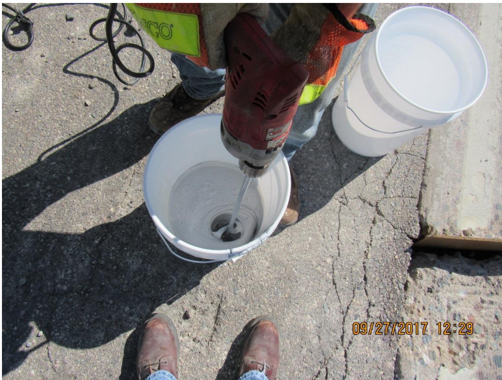
Photograph: 94004 D.S. Brown, PaveSaver Polymeric Concrete
