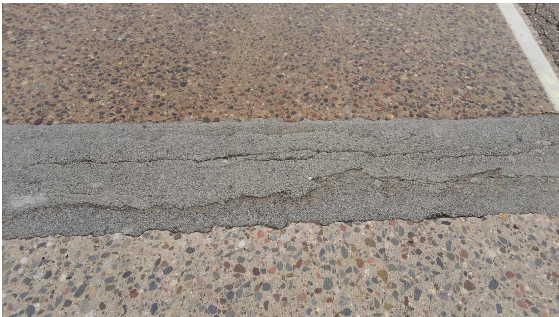
Figure 5.28 Cell 94009 – General condition, cracking (Rating – 3)
