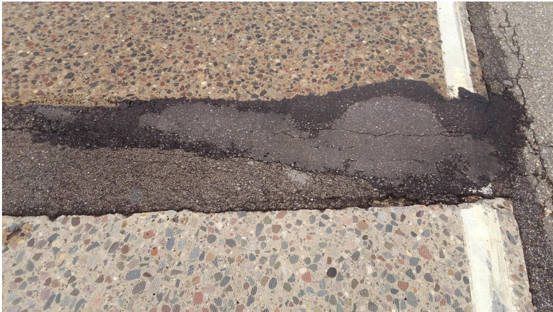
Figure 5.6 Cell 94002 (B) – General condition, linear cracks and repairs (Rating – NA)
