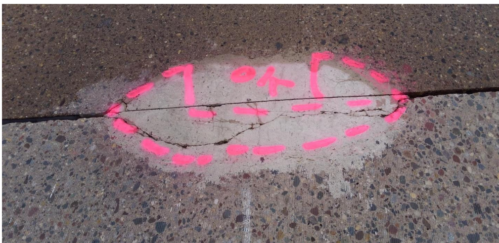
Figure 5.36 Cell 94013 (A) – General condition, cracking and debonding (Rating – 3)
