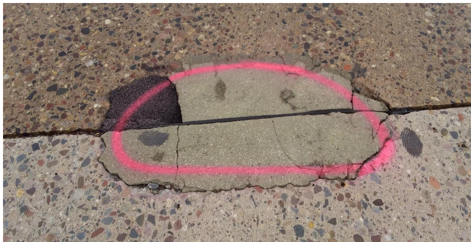
Figure 5.18 Cell 94006 (A) – General condition, cracks, debonding and loss (Rating – 2)
