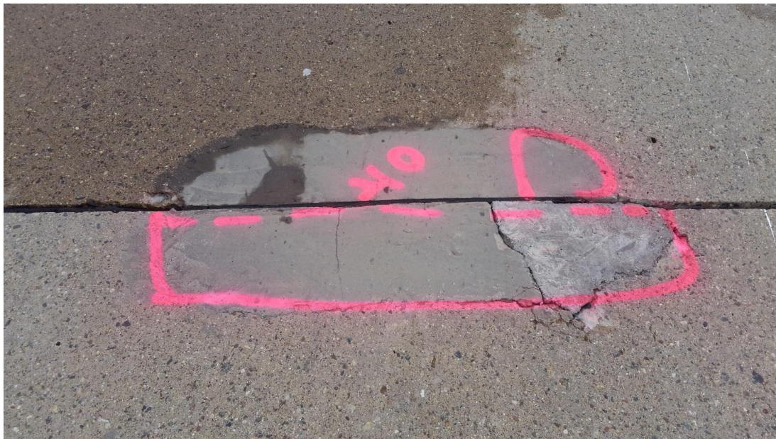
Figure 5.22 Cell 94007 – General condition, cracks, debonding, and loss (Rating – 2)
