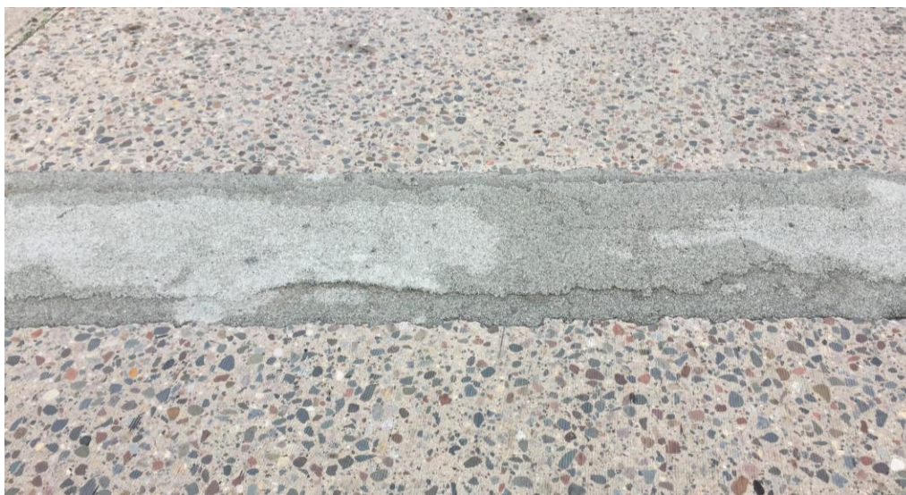
Figure 5.22 Cell 94009 – General patch condition (Rating – 4)
