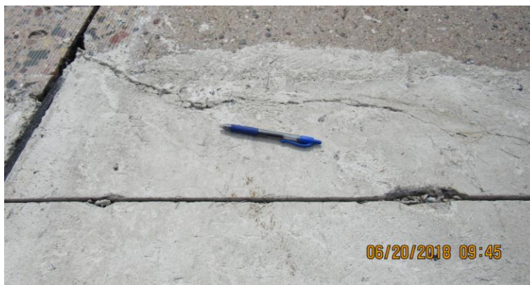
Figure 5.30 Cell 94013 (A) – WP patch, cracking along edge (Rating – 3)
