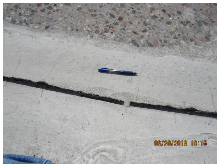
Figure 5.2 Cell 94001 – General patch condition, minor shrinkage cracks (Rating – 4)
