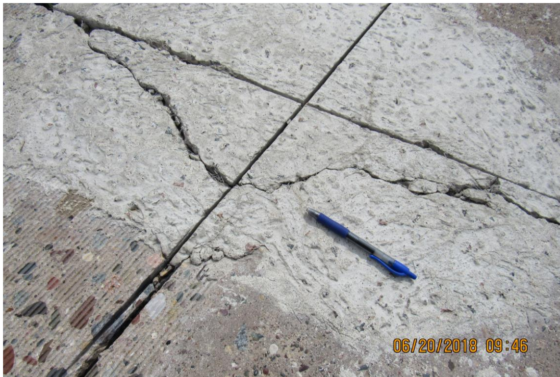
Figure 5.32 Cell 94013 (B) – CLJ patch, cracking near edge (Rating – 3)
