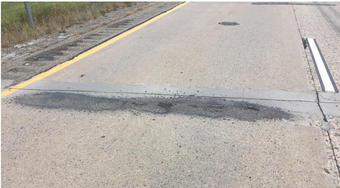
Figure 5.20 Cell 94008 (B) – General condition, cracks and missing material (Rating – 2)
