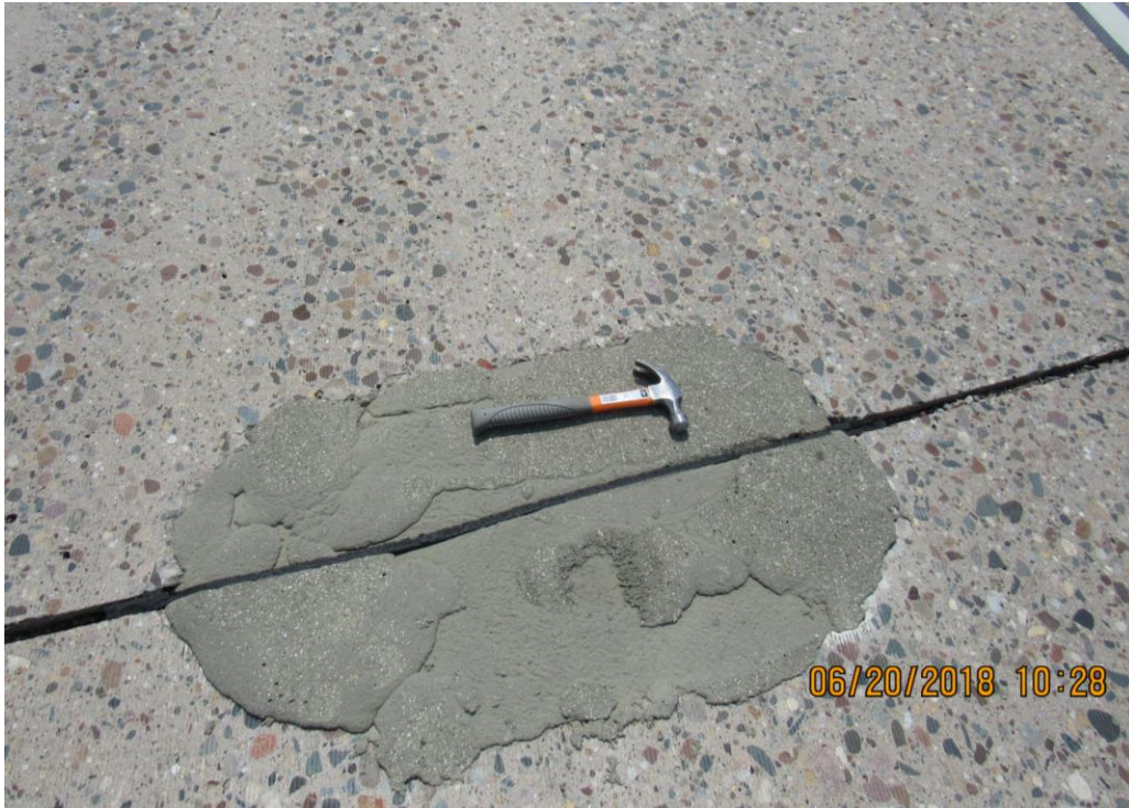
Figure 5.12 Cell 94006 (A) – General patch condition (Rating – 4)
