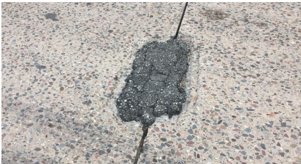
Figure 5.18 Cell 94008 (A) – General condition, cracks and missing material (Rating – 2)
