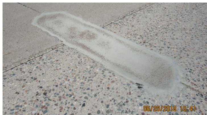
Figure 5.24 Cell 94010 – General patch condition (Rating – 4)
