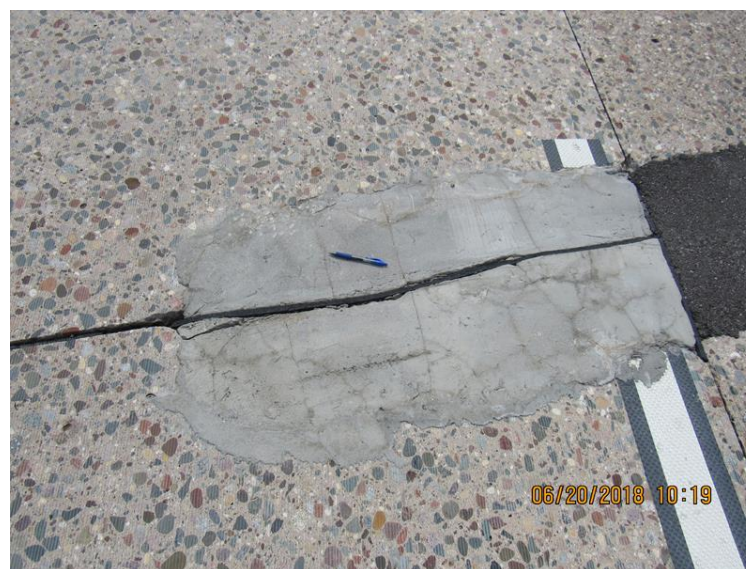
Figure 5.4 Cell 94002 (A) – General patch condition, linear cracks present (Rating – 3)
