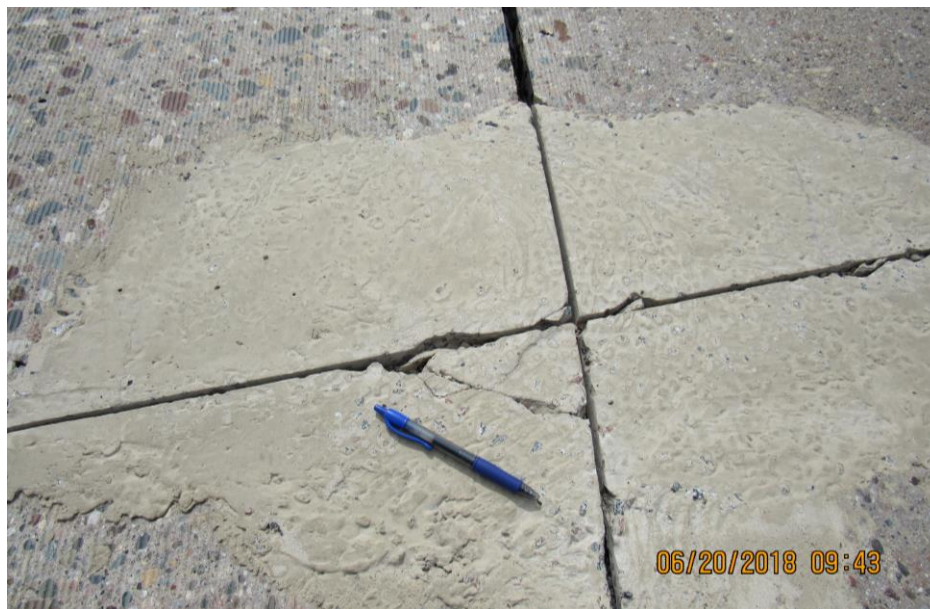
Figure 5.28 Cell 94012 – CLJ patch, corner break and cracking (Rating – 3)
