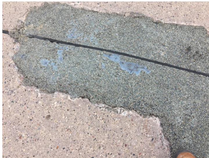
Figure 5.14 Cell 94006 (B) – General patch condition, minor cracks and debonding (Rating – 3)
