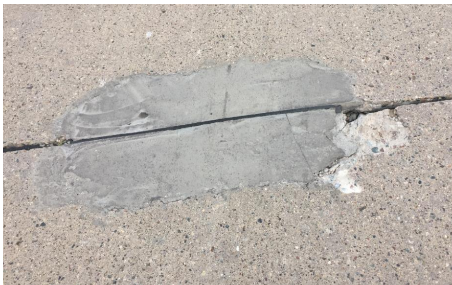
Figure 5.16 Cell 94007 – General condition, minor cracks and missing material (Rating – 2)
