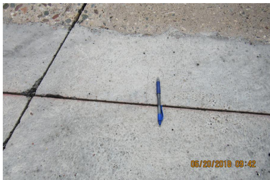
Figure 5.26 Cell 94011 – General patch condition (Rating – 4)
