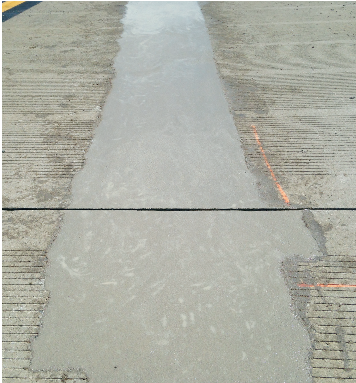
PaveSaver™ Airfield Repair Application
