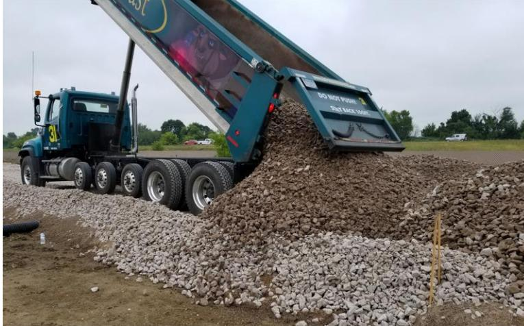
**Figure 2.4. Placement of LSSB material (White and Vennapusa 2017)**
