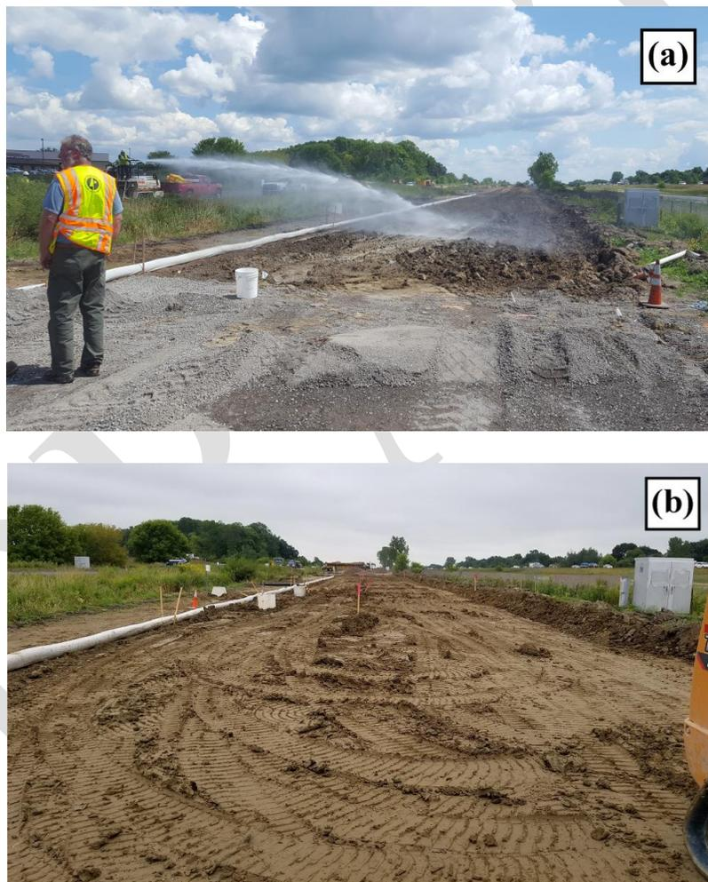
**Figure 2.3. (a) Moisture content adjustment for subgrade soil and (b) prepared subgrade (White and Vennapusa 2017)**
