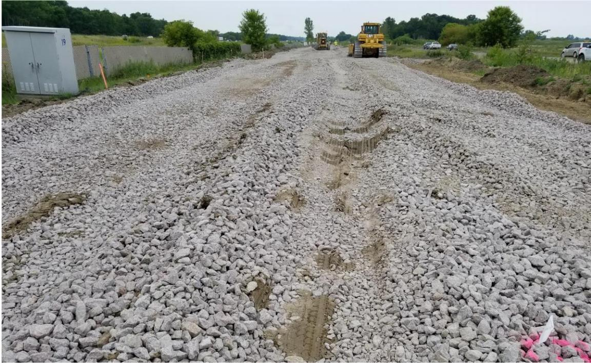
***Rutting on LSSB layer and subgrade soil pumping under construction traffic (White and Vennapusa 2017):***
