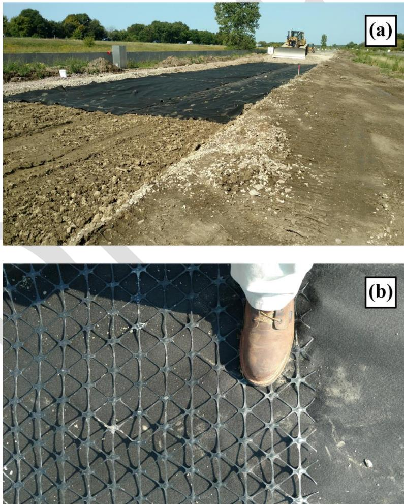
**Figure 2.8. Placement of (a) geotextile and (b) triaxial geogrid over geotextile (White and Vennapusa 2017)**
