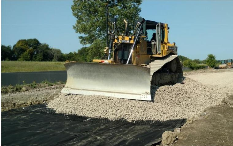
**Figure 2.9. Placement of LSSB material over geosynthetics (White and Vennapusa 2017)**
