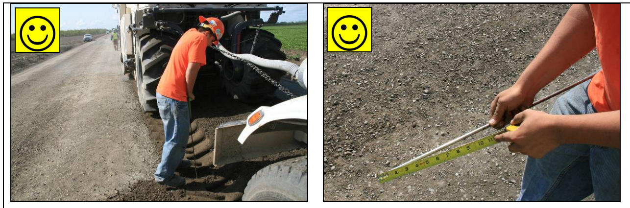
Figure 7.5: Checking mixing depth.
