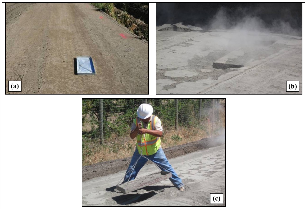
Figure 7.4: Monitoring stabilizer application rate.
