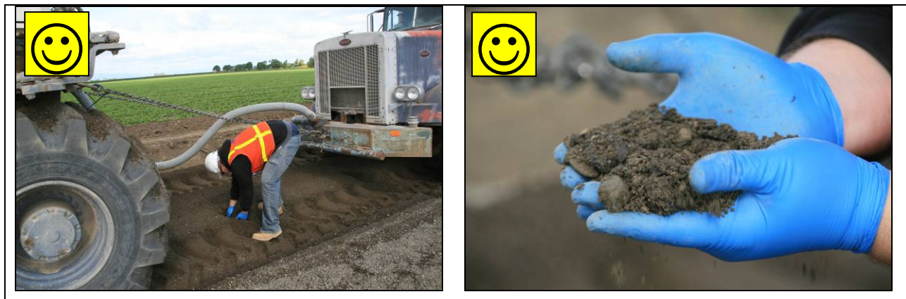
Figure 7.6: Checking material consistency and color.
