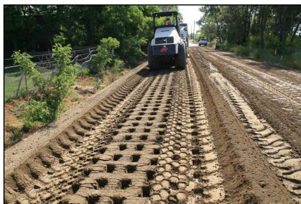
Figure 7.11: First padfoot roller pass impressions.
