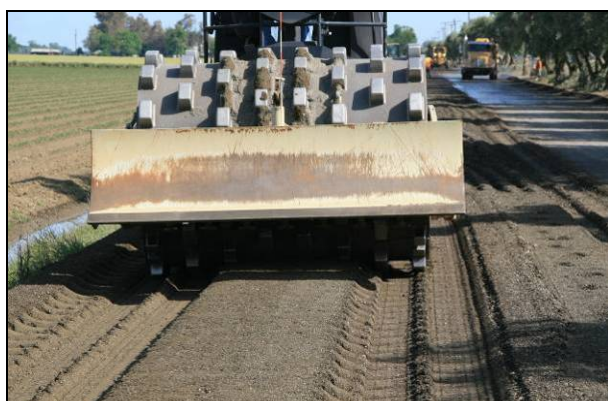
Figure 7.9: First padfoot roller pass.
