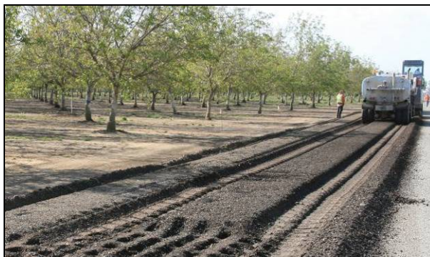
Figure 7.8: Differential compaction in rotary mixer/recycling train wheelpaths.
