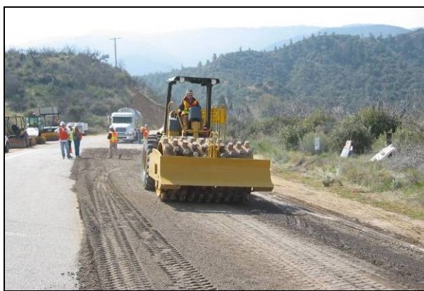
Figure 7.12: Padfoot impressions after multiple passes.
