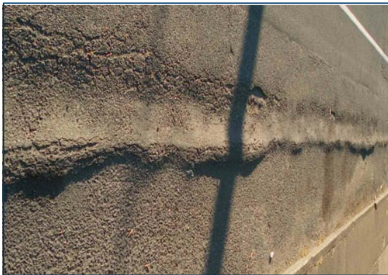
Rutting failure due to the weak shear strength of subgrade
