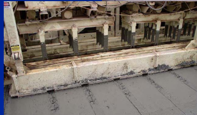
Dowel Bar Insertion
